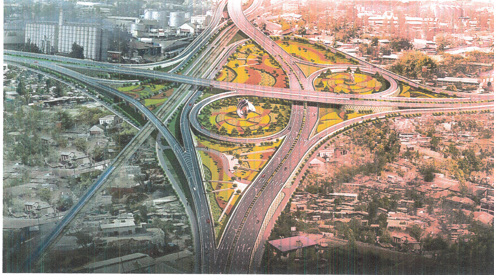
GOTERA INTERCHANGE (UNDER CONSTRUCTION)
