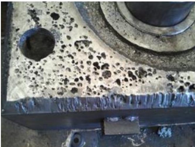
(c) Blow holes
