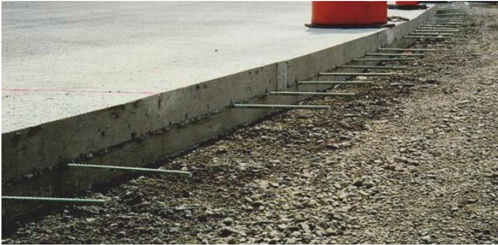
Figure 2-1: Tie bars in place to connect to parallel concrete slab
