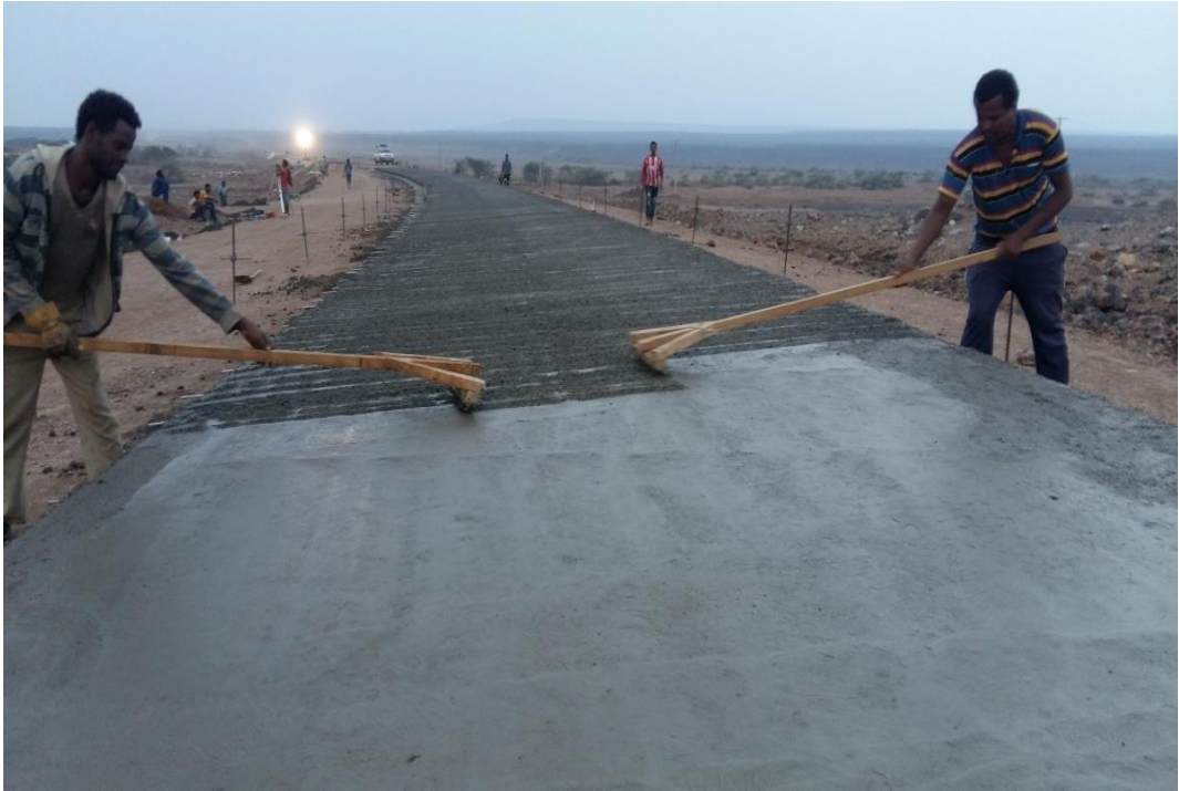
Traverse oriented surface texturing using wire or plastic broom
