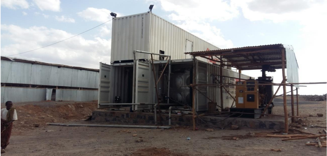
Chiller plant cap. 100,000 lit ~ up to 1 oC
