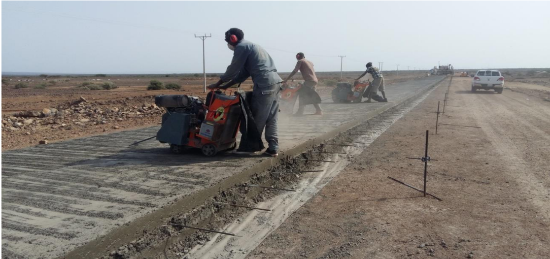
Joint Cutting Activity
