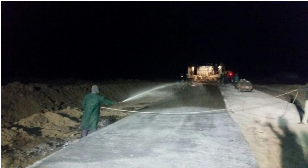
Traverse oriented surface texturing using wire or plastic broom
