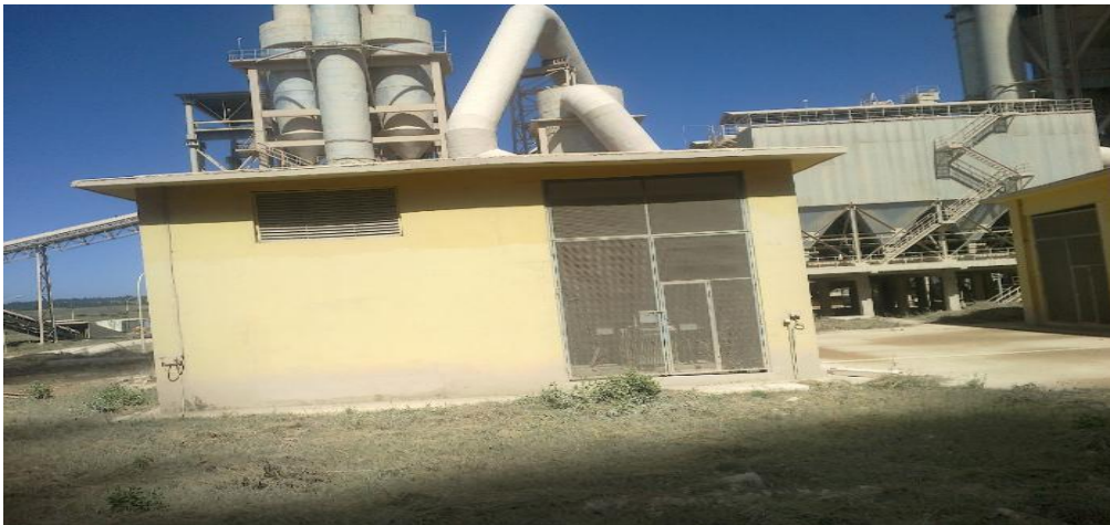
Figure 4.20: Generator set building (Source: Picture taken on site)
