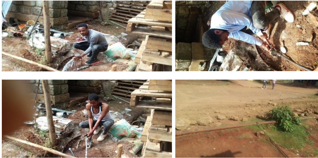
Figure 12: Sample measured junction pressure data validation and time series with distribution network
