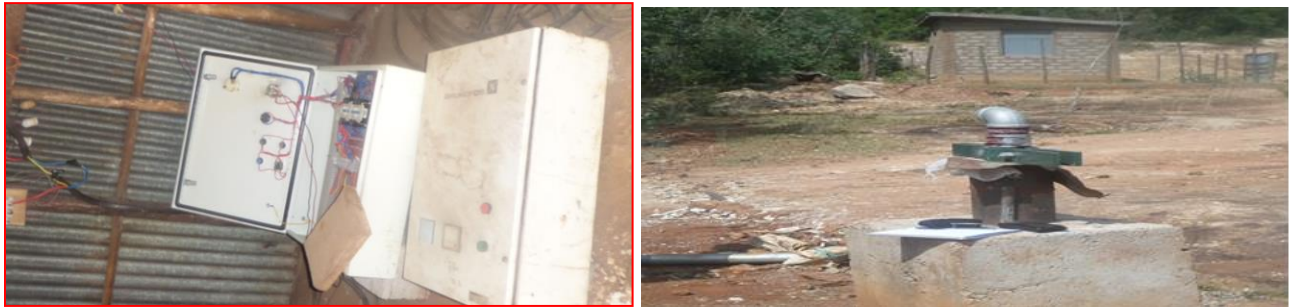
Figure 7: Existing pump station and newly drilled borehole
