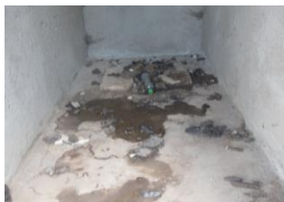
PPS-3 (common latrine)
