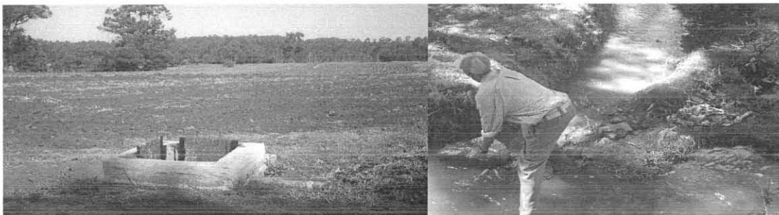
Figure 5. Holetta research center open and closed channel for irrigation
