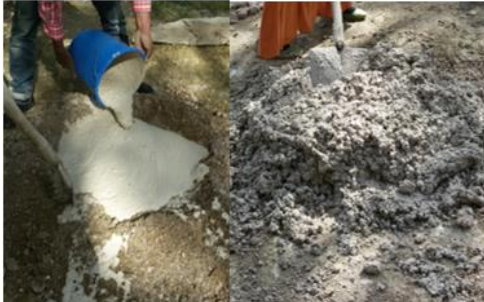
Figure 3.3 Mixing of aggregate with the lime putty and prepared mortar
