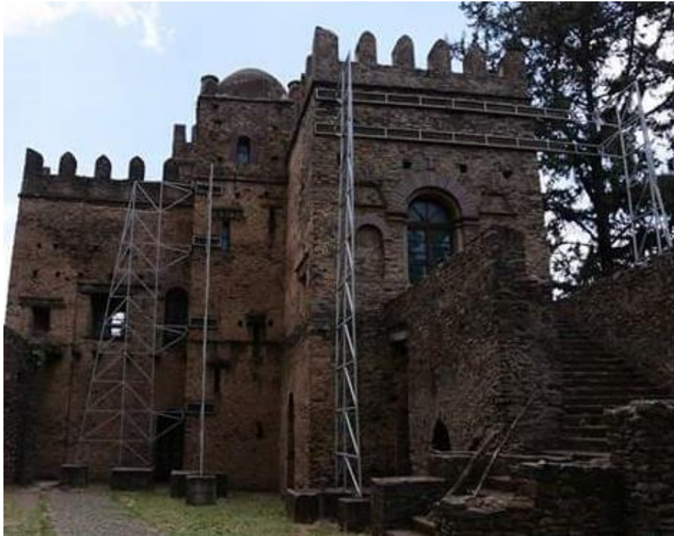
Figure 5.6 Shoring on the east and south of the castle
