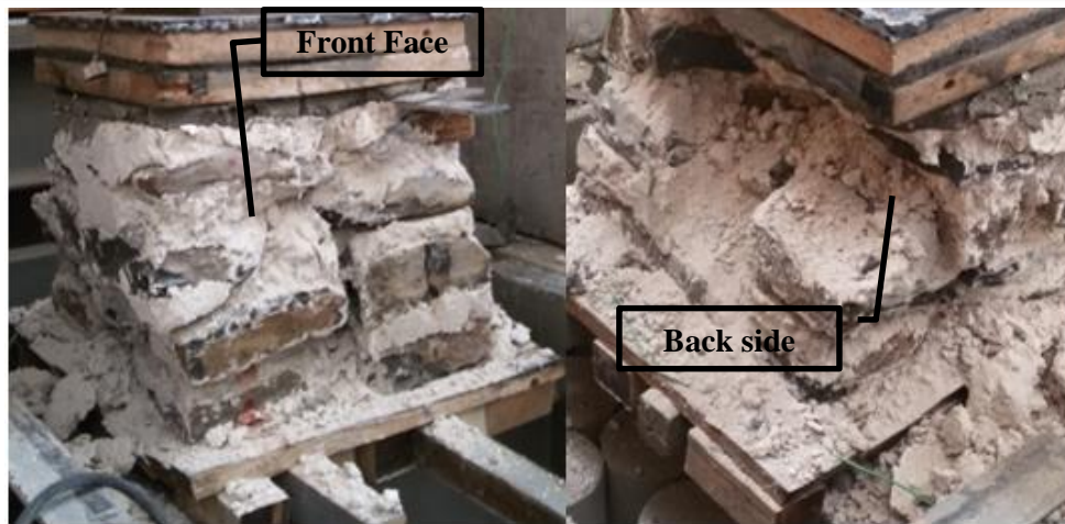
Figure 4.11 Specimen C1 after compression test (failure mode)
