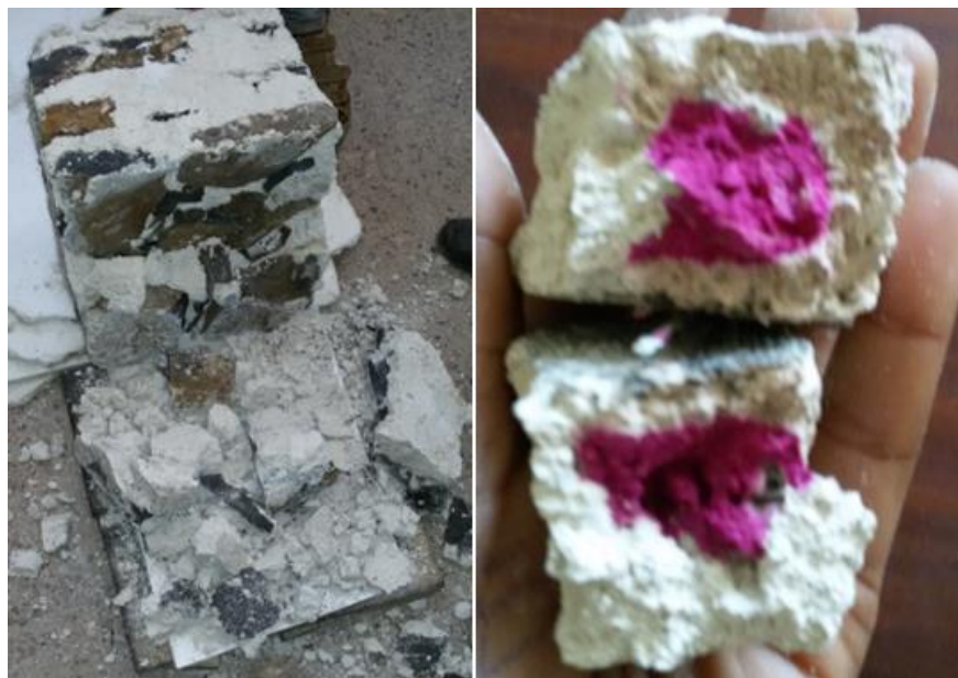
Figure 3.16 Broken specimen and phenolphthalein test on the mortar
