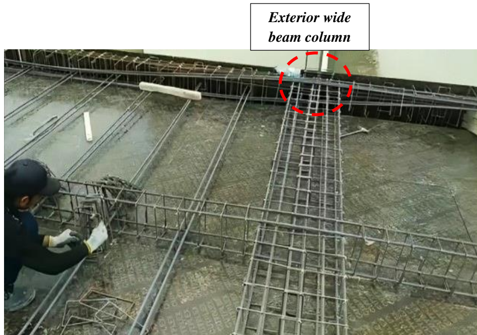
Figure 2- 1 Exterior RC wide beam column joint
