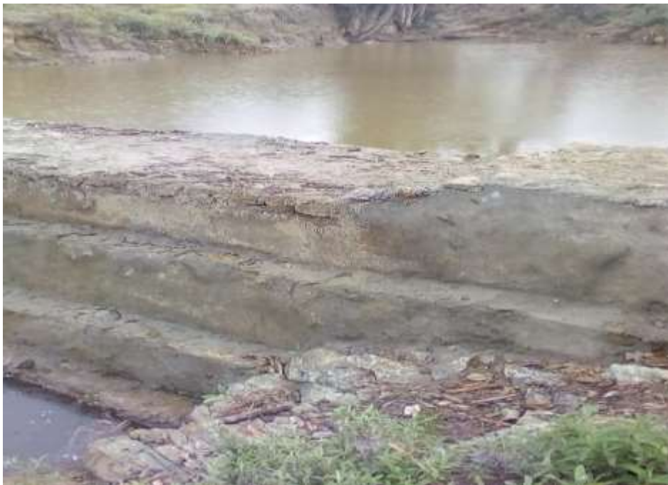
Figure 8: Small scale dam in Biera
