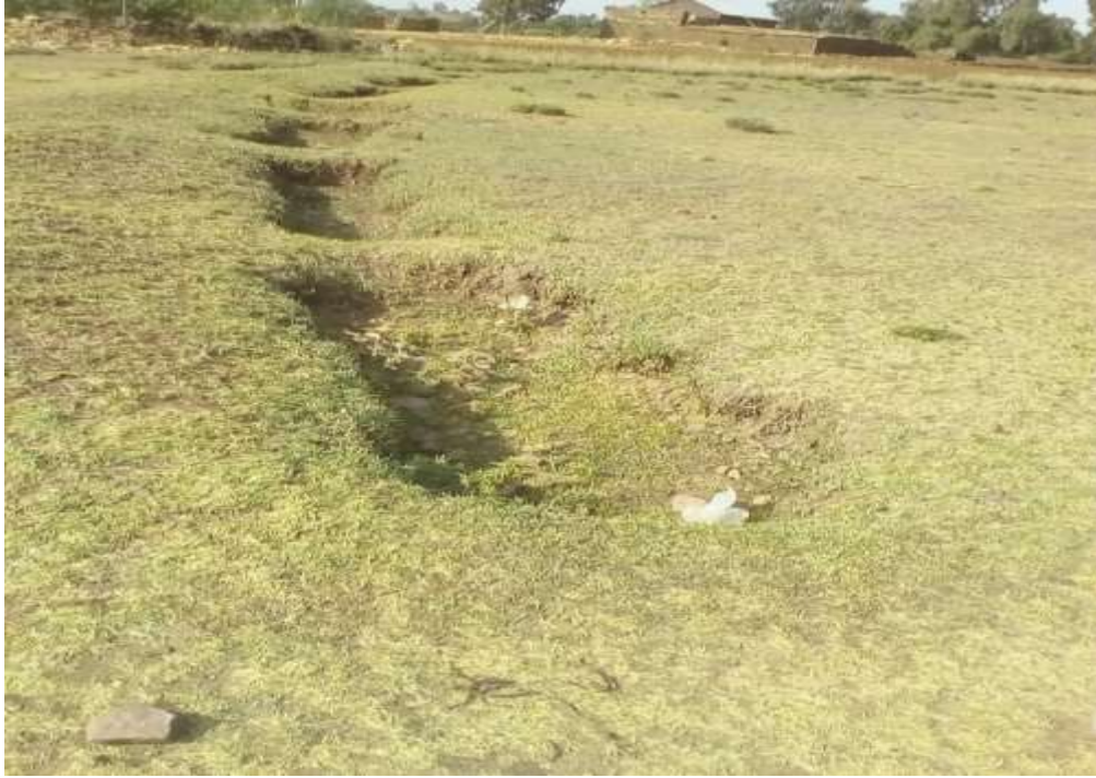
Hand-dug trenches Method of SWC in Kebelle Saesie
