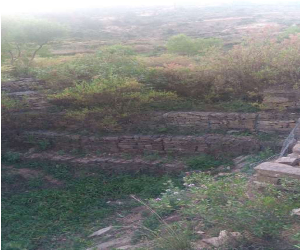
Figure 7: Check dam in Awleat
