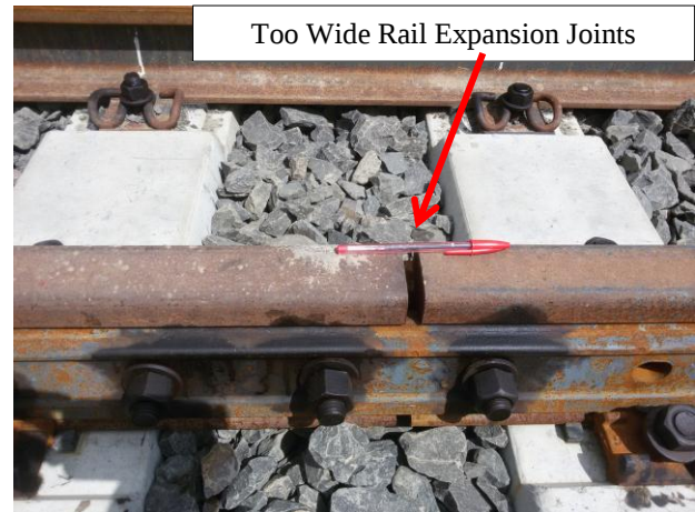
Too Narrow and Too Wide Rail Expansion Joints, Around Alemgena ERC
