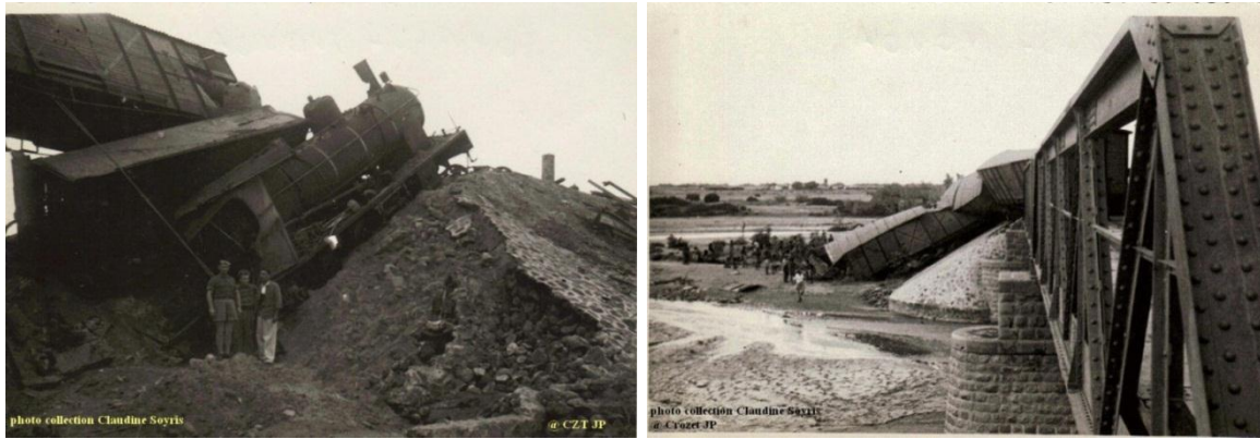
Figure 2-15: Train Accident due to Bridge Abutment scoured 1935 [22]
