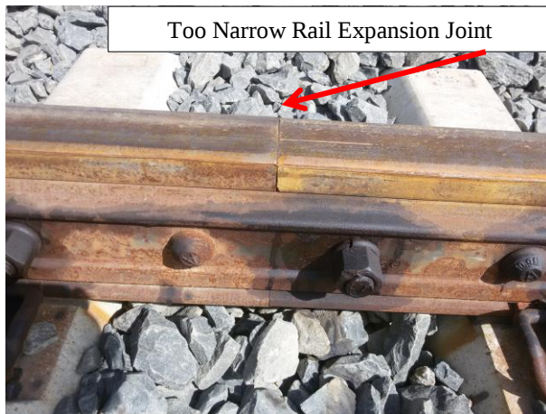
Too Narrow and Too Wide Rail Expansion Joints, Around Alemgena ERC
