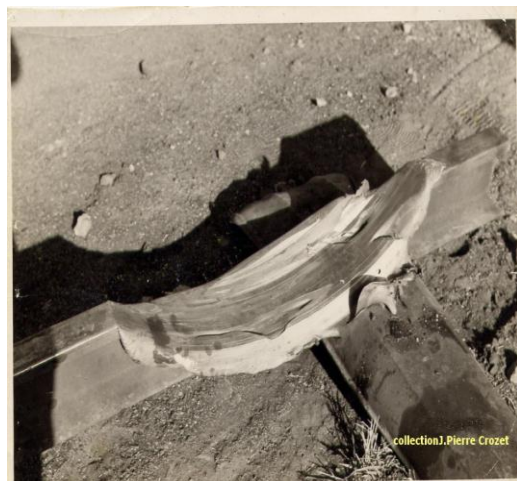
Deformation of rail, Ethio-Djibouti Railway Line 1964 [22]
