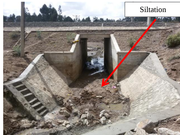
Water way Scour and Siltation on Bridge around Alemgena, ERC
