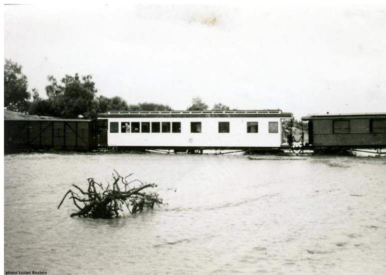
Figure 2-19: Oued Andobed Bridge 1950 [22]
