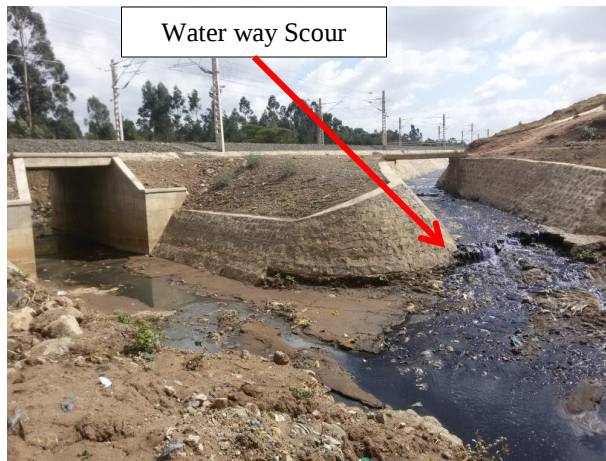
Water way Scour and Siltation on Bridge around Alemgena, ERC
