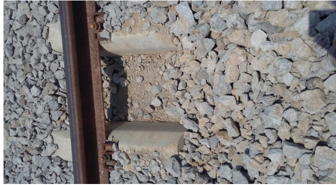
Dust and silt on railway track. [23]
