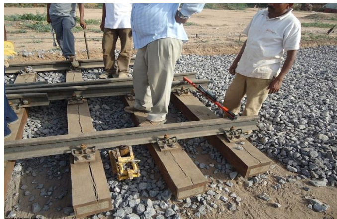
Level & Gauge Checking around Metehara (Beseka Lake) during the rehabilitation of Ethio-Djibouti Railway Line [22]
