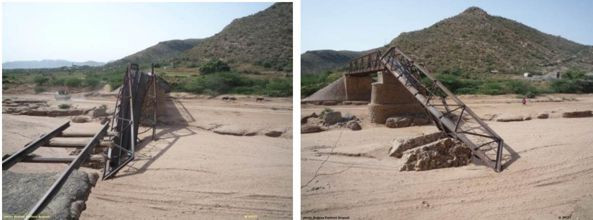
Figure 2-14: Laga Oda Bridge [22]
