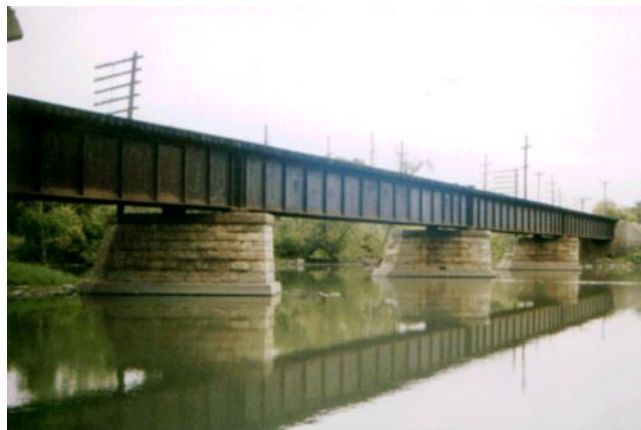
Figure 2-7: Deck Plate Girder [17]
