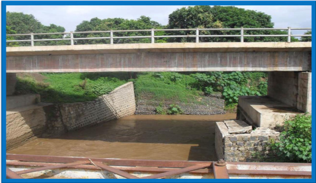
Photo1-7: Right Bank with Protection Work (Source: ERA-BMS, August 2012)
