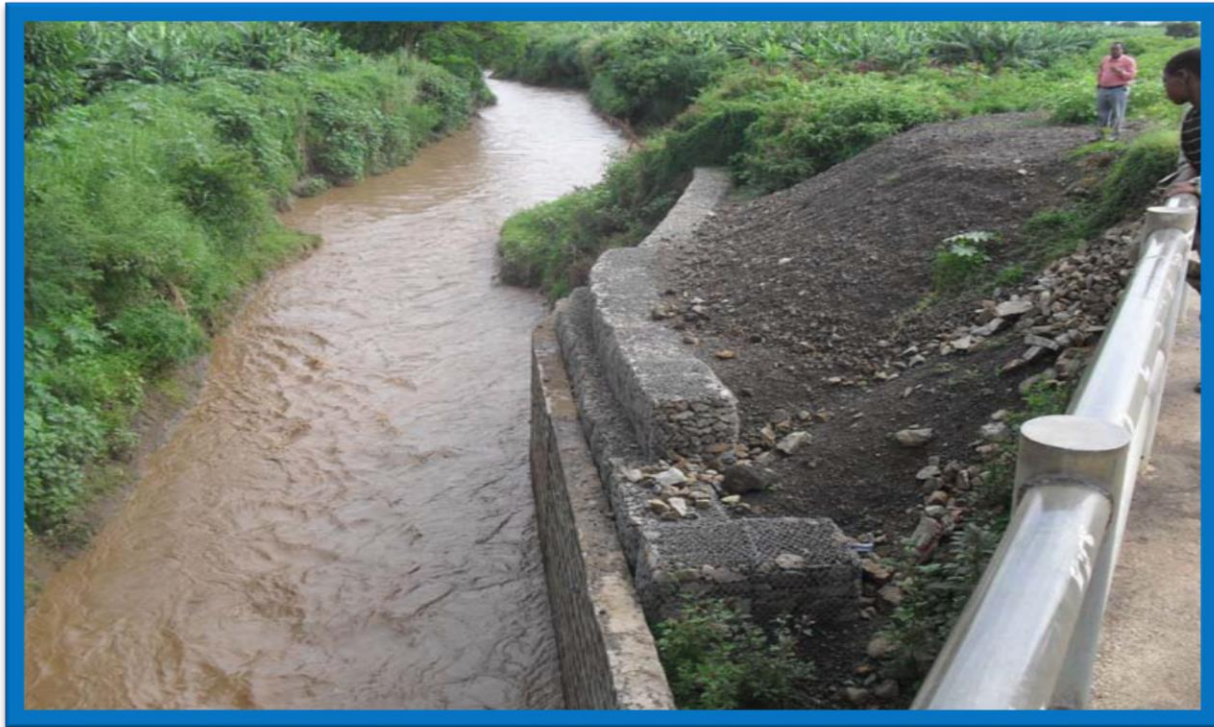
Photo1-5: Left Bank with Embankment Protection (Source: ERA-BMS, August 2012)
