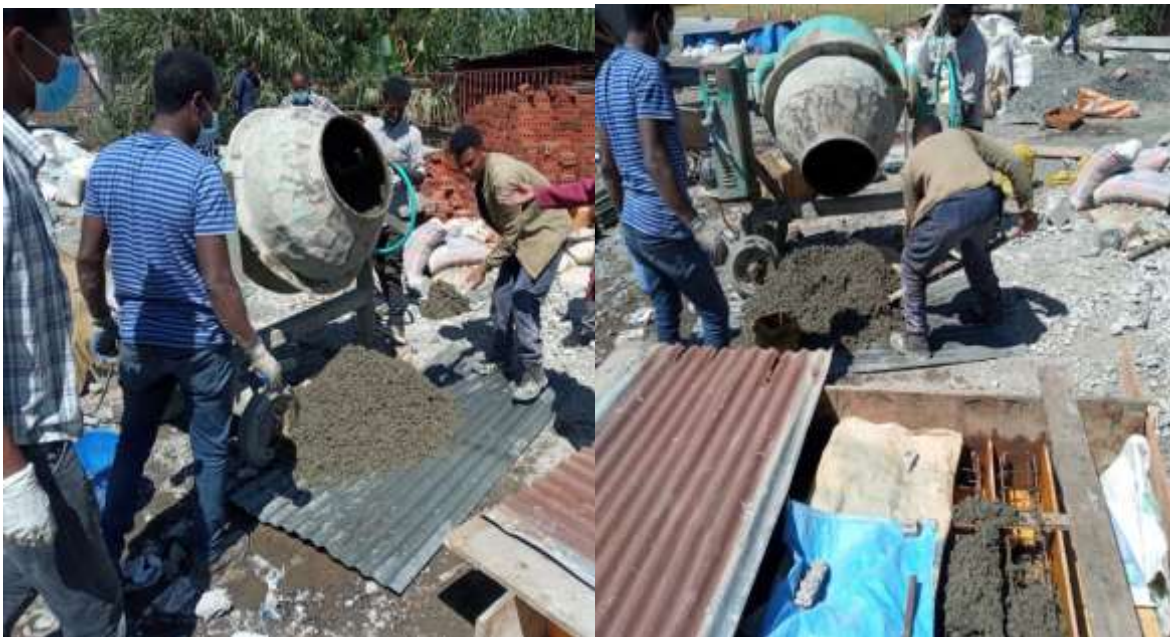
Figure 3.5 concrete mixing and cylinder, cube, and flexure taken
