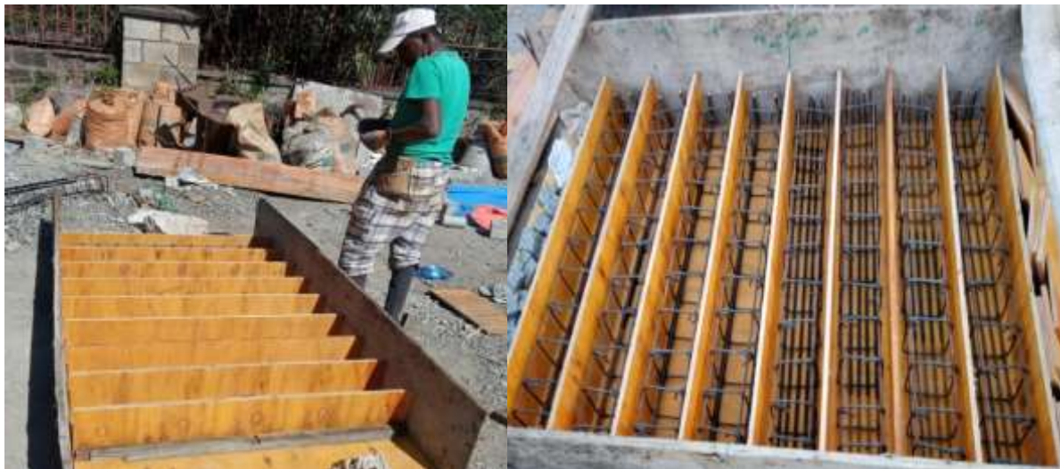
Figure 3.9 Plywood formwork preparations
