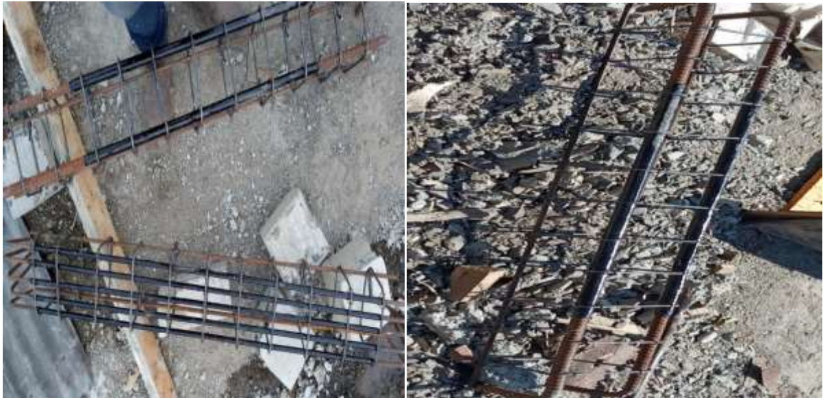
Figure 3.11 Preparation of unbounded reinforcement specimen
