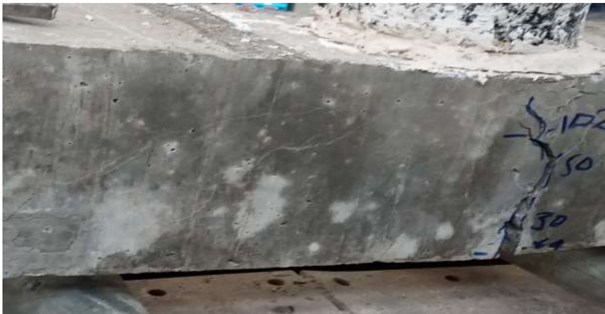
Figure 4.2 Flexural failure of specimen B22
