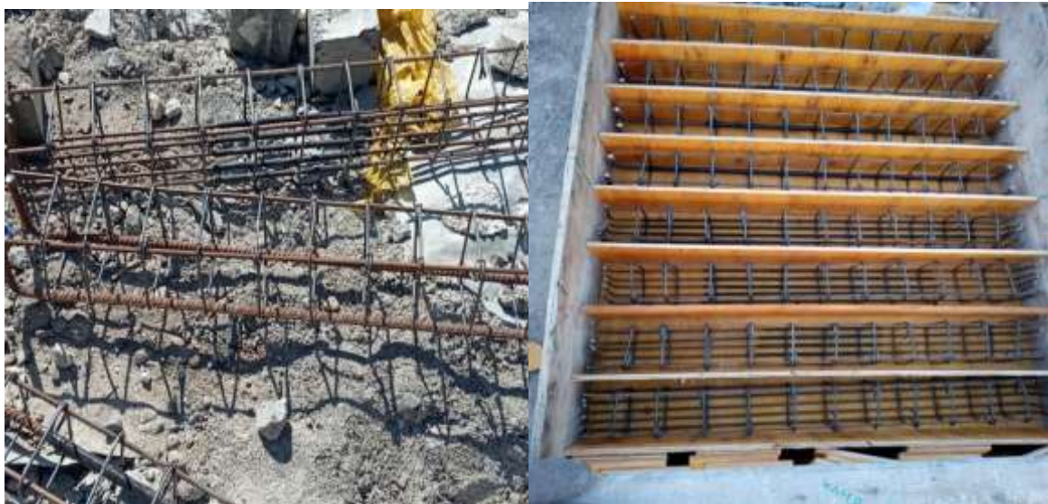
Figure 3.10 Specimen reinforcement preparations
