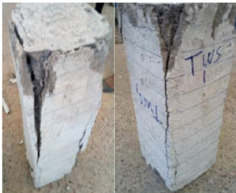
Figure 5-12: Typical failure pattern TWSC
