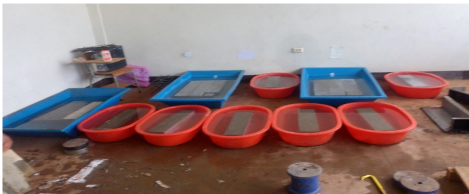
Figure 3-13: Curing the strengthened column
