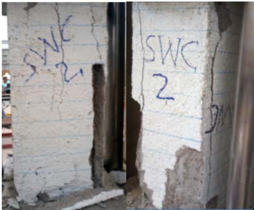
Figure 5-10: Typical failure pattern SWCS
