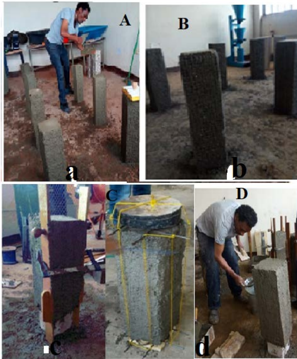
Figure 3-12: Strengthening procedure (a) applying first coat (b) wrapping mesh wire (C) keeping horizontal and vertical alignment (d) finishing
