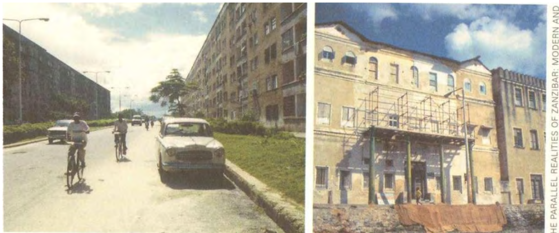
Figure 3-19: Some Buildings in the Town of the Case Review, from Battle, Melin, and Forsman 2007
