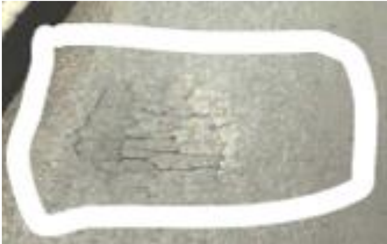
Figure 2- 3 block cracking
