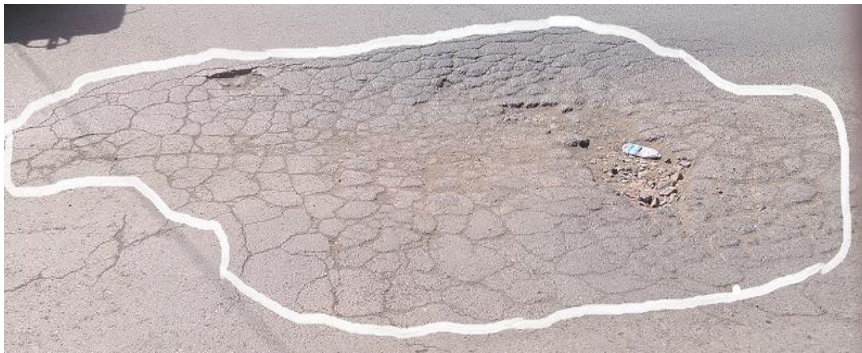
Figure 2- 2 fatigue cracking
