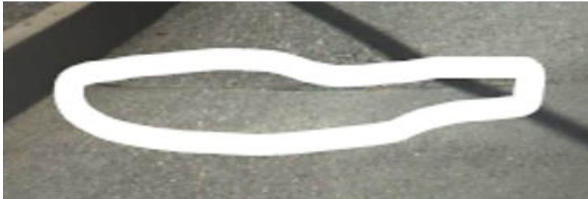
Figure 2- 4 transverse cracking
