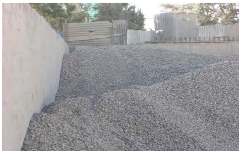
Figure 2.7 handling of aggregates around the concrete batching plant (Admasu, 2015)
