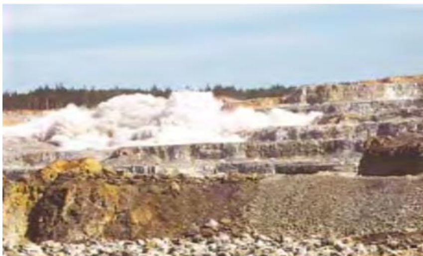
Figure 2.10 rock drilled and blasted as crushed stone (Langer, et al., 2001), as cited in (Semere, 2013)
