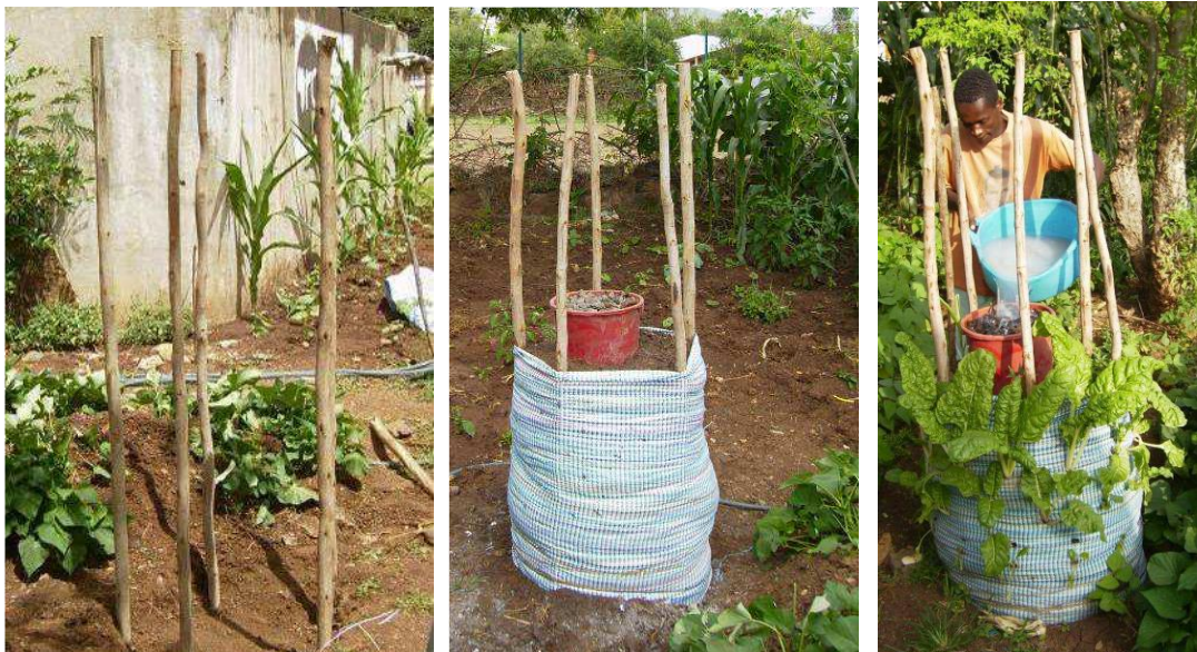
Figure 2-7 Process of making Greywater Tower
