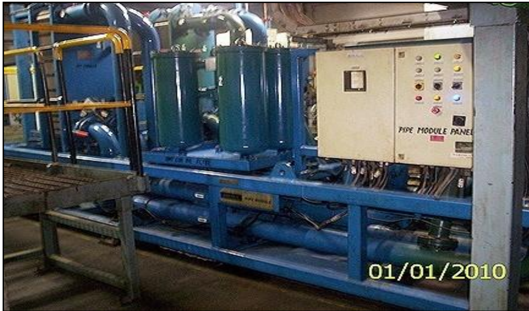
Figure 17 4.2MW Wartsila HFO Power Plant
