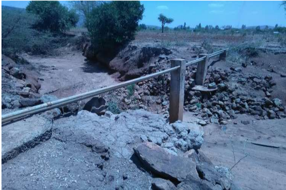
Figure 14: Pressure Pipeline Changed with two parallel pipes
