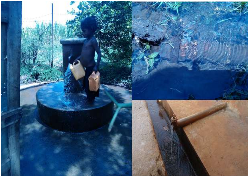
Figure 18: Photo shows losses. (Source: Own field visit photo)
