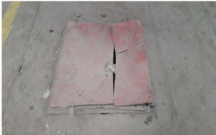
Figure 4.17: Metallic manhole cover used in the case company
