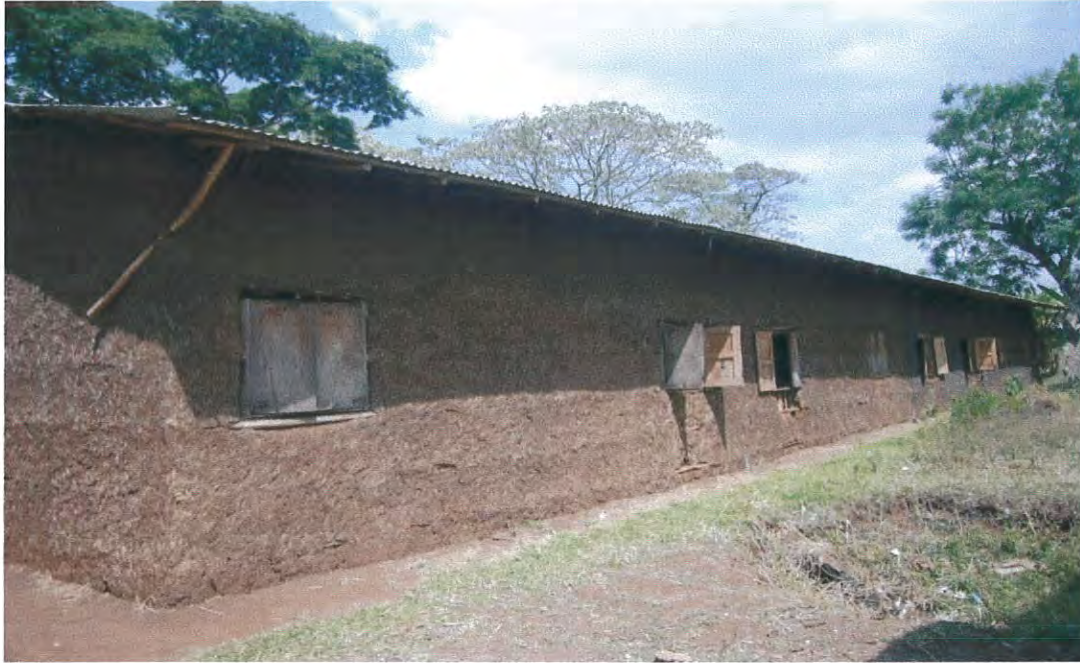
Figure 14: School expansion to Haro elementary school, Haro cooperatives
