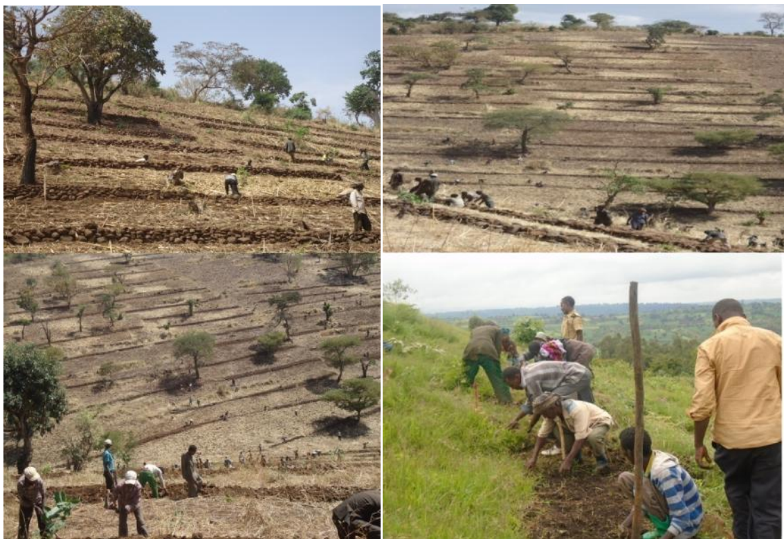
Figure 7: Stone terrace development in Metu Sillasie of Nono Woreda, (three pictures from left to right). Development's of grass strip in Gololle kebele of Nono Woreda (right end). Source: Field survey.
