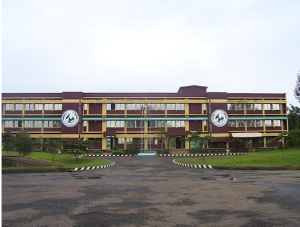
Figure 9. Bedele Brewery Main Office Block after immediate Main Entrance.
