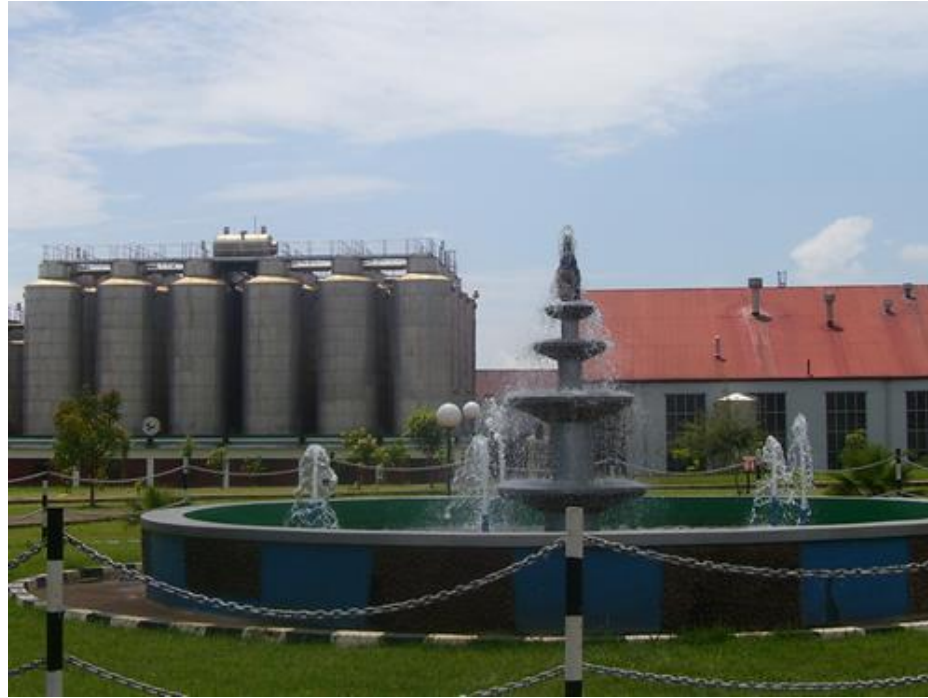
Figure 10: Bedele Brewery Fountain & beer processing unit tank.
