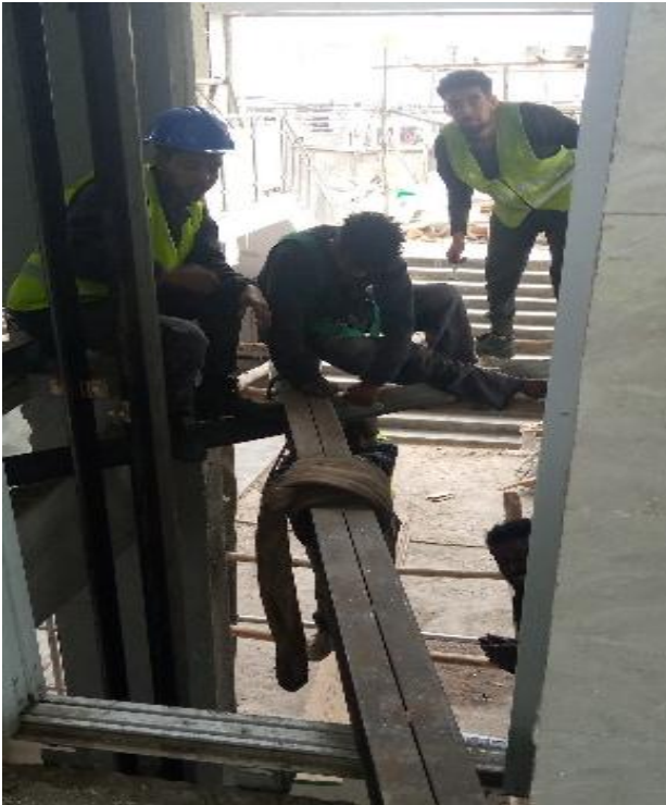
Figure 4.2: Shows how employees working at 50m height without keeping safety procedure and safety equipment observed on site.
