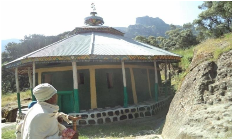
Fig.3.10 The church of Abäkäna Abbo, north-western side
