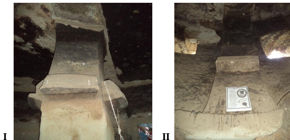
Fig.3.8 (I) A doubled layered pillar; fig.3.8 (II) a pilaster on the wall of the church
