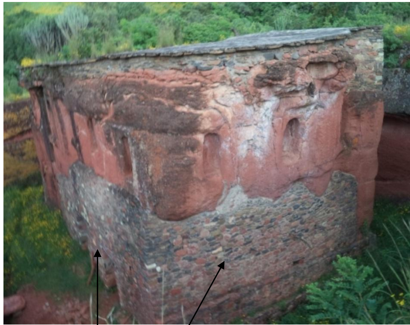
Fig. 3.13 Northern and western facade of Nazugn Maryam church
