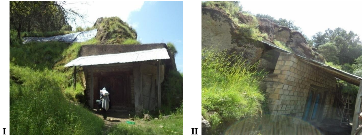
Fig. 3.15(I) Eastern side of the church; fig.3.15 (II) western side of the church
