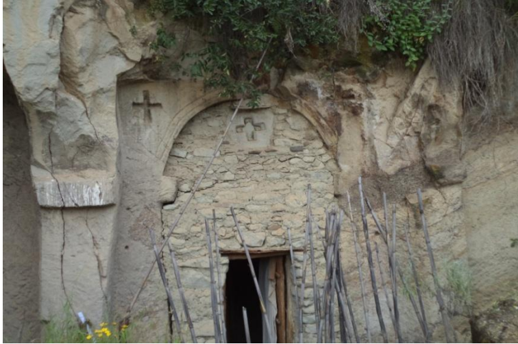
Fig.3.19 The arch shaped, frieze decorated and crosses engraved entrance in to the gəbə'atä mänṭola'et
