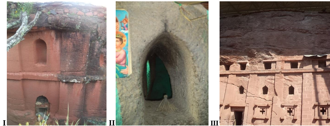
Fig.4.2 shapes of windows at the churches of Nazugn Maryam (I), Abäkäna Abbo (II) & Bétä Abba Libanos in Lalibela(III), note the pointed features at the top-mid part of the windows
