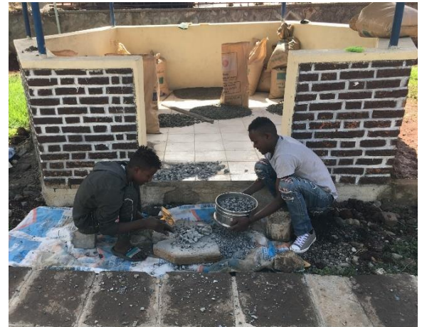
Figure 3-10: Crushing of recycled aggregates using different kinds of hammers
