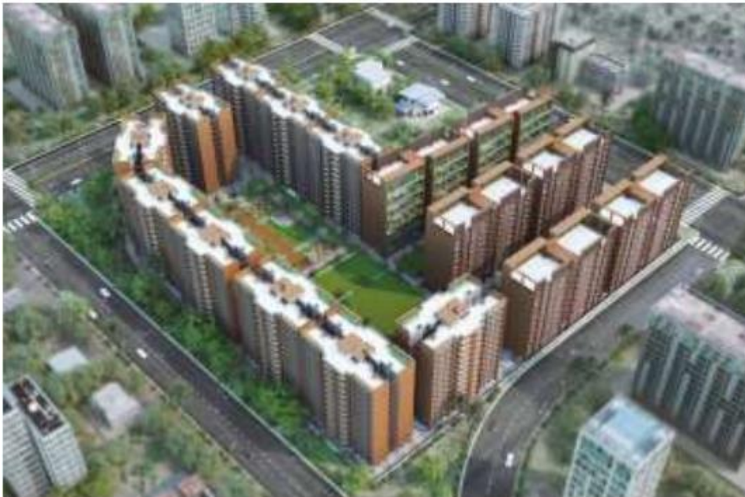
Figure 3. Gerji higher official housing project. (Zinabu, 2022)
