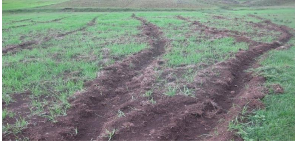
Figure 9: Cutoff drains in Kata Walele (Field Survey, 2014)
