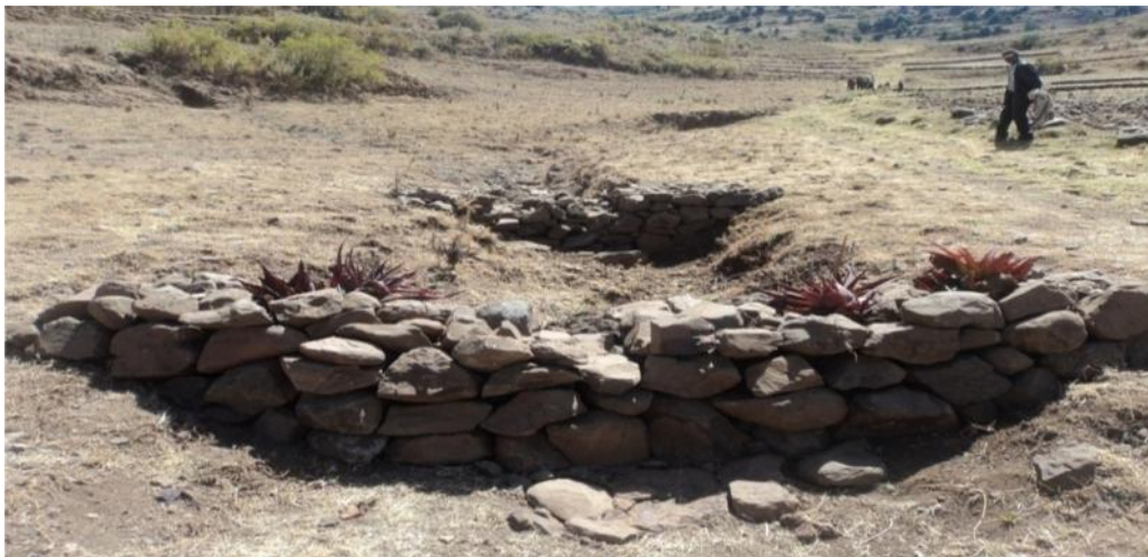
Figure 10: Photo shows gully rehabilitation in Warerso Malima (Field Survey, 2014).
