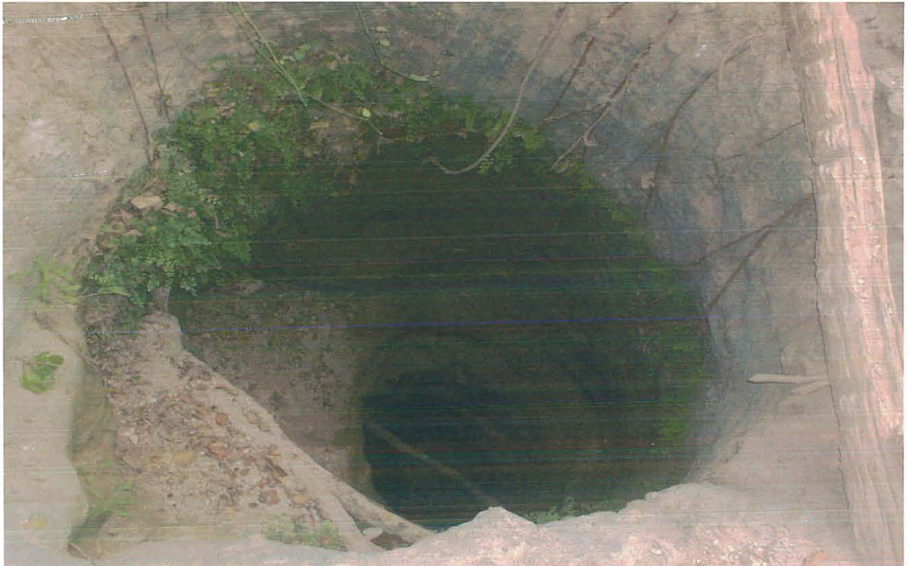
Figure 10. Deep walls ( Tulla ) estimated to 30 meter depth
