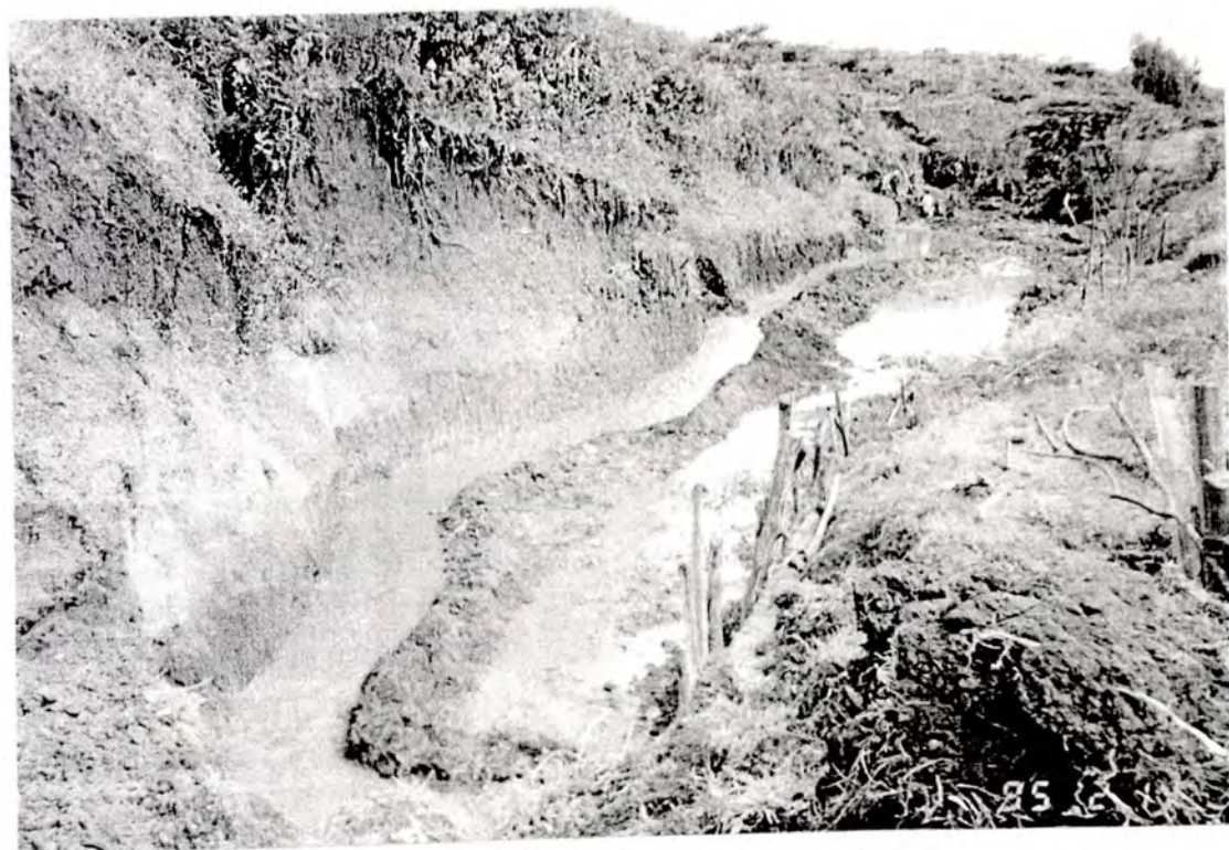
Plate: 4 The Maintained Channel
