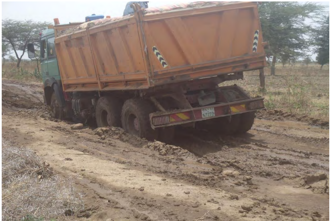
Fig 2.5 A Truck with sand in deteriorated access road around Alemtena.
