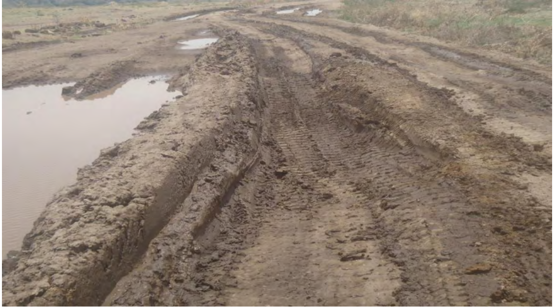
Fig 2.6 Deteriorated access road around Alemtena to sand source.
