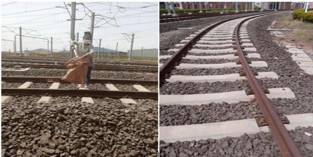
Figure 6: Railway line at Kality Depot
