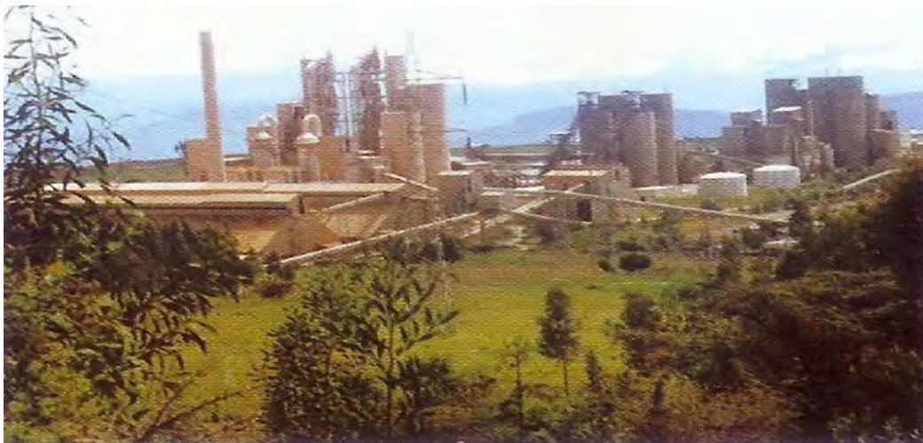
Fig. 2.2 Mughar cement plant [20]
