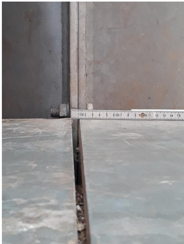
Figure 3.1.1-9:-Column-D1 (It's been witnessed that different width of openings occurred on the base plates in four direction) (photo by Naol G.).
