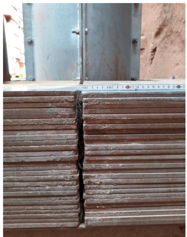
Figure 3.1.1-9:-Column-D1 (It's been witnessed that different width of openings occurred on the base plates in four direction) (photo by Naol G.).
