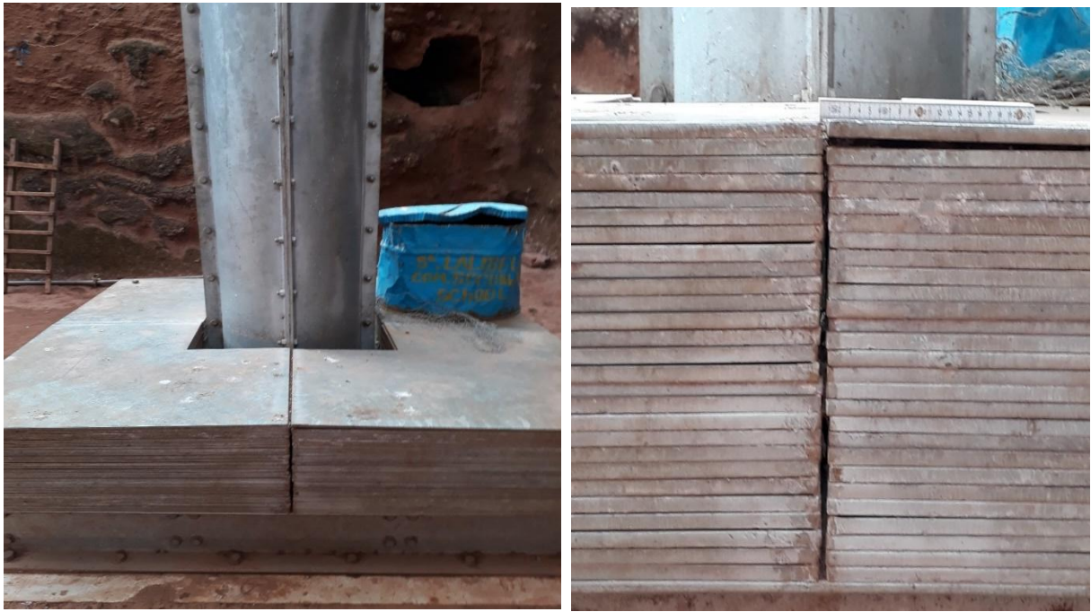
Figure 3.1.1-11:-Column-D3 (Bending of plates towards the column center and Slight uniform opening of plate is witnessed on this column)
