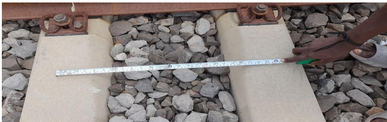
Figure 3.5: Sleeper placement with 600mm spacing as measured at the actual site
