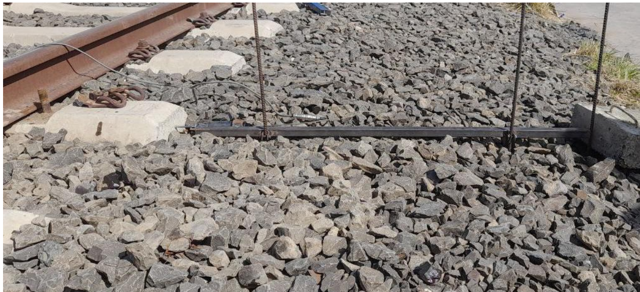
Figure 3.13: Installation of the transducer on the tested sleeper using support fixtures
