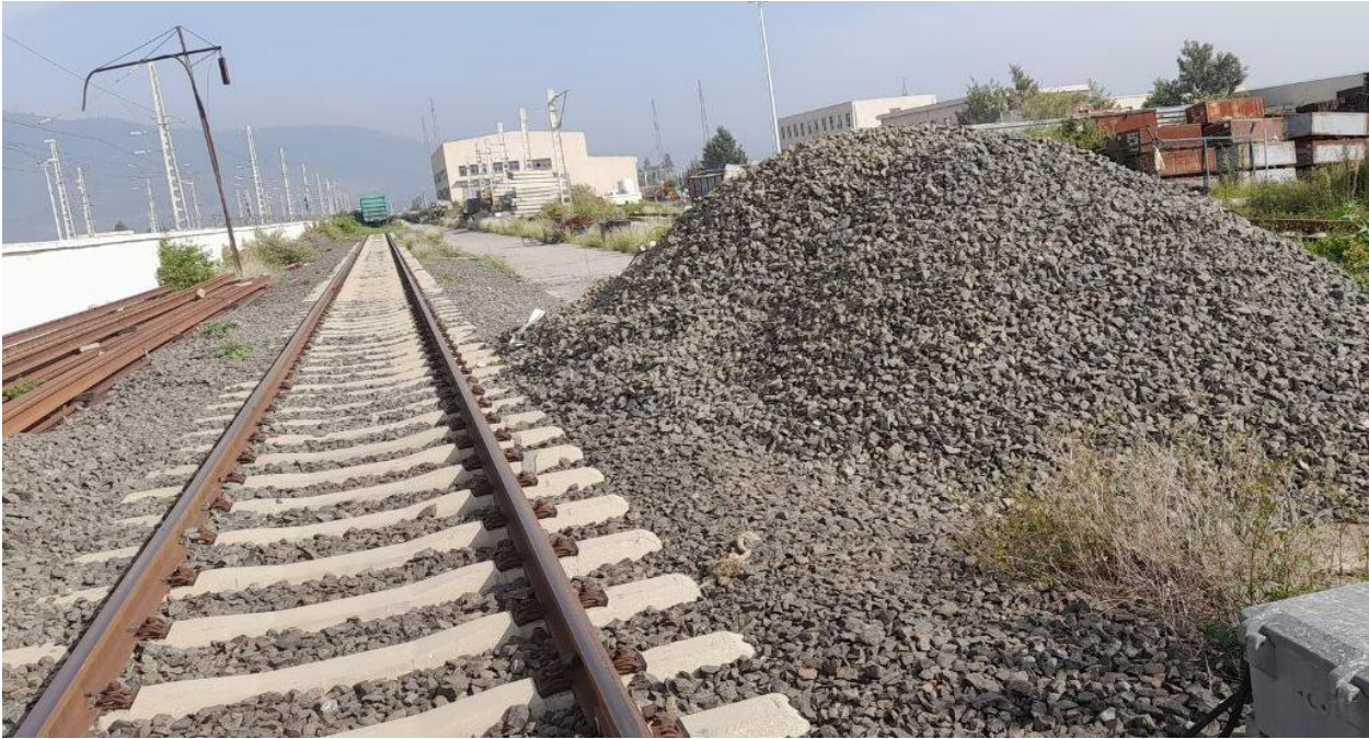
Figure 3.2: Tested sub- track line at Indode Railway station
