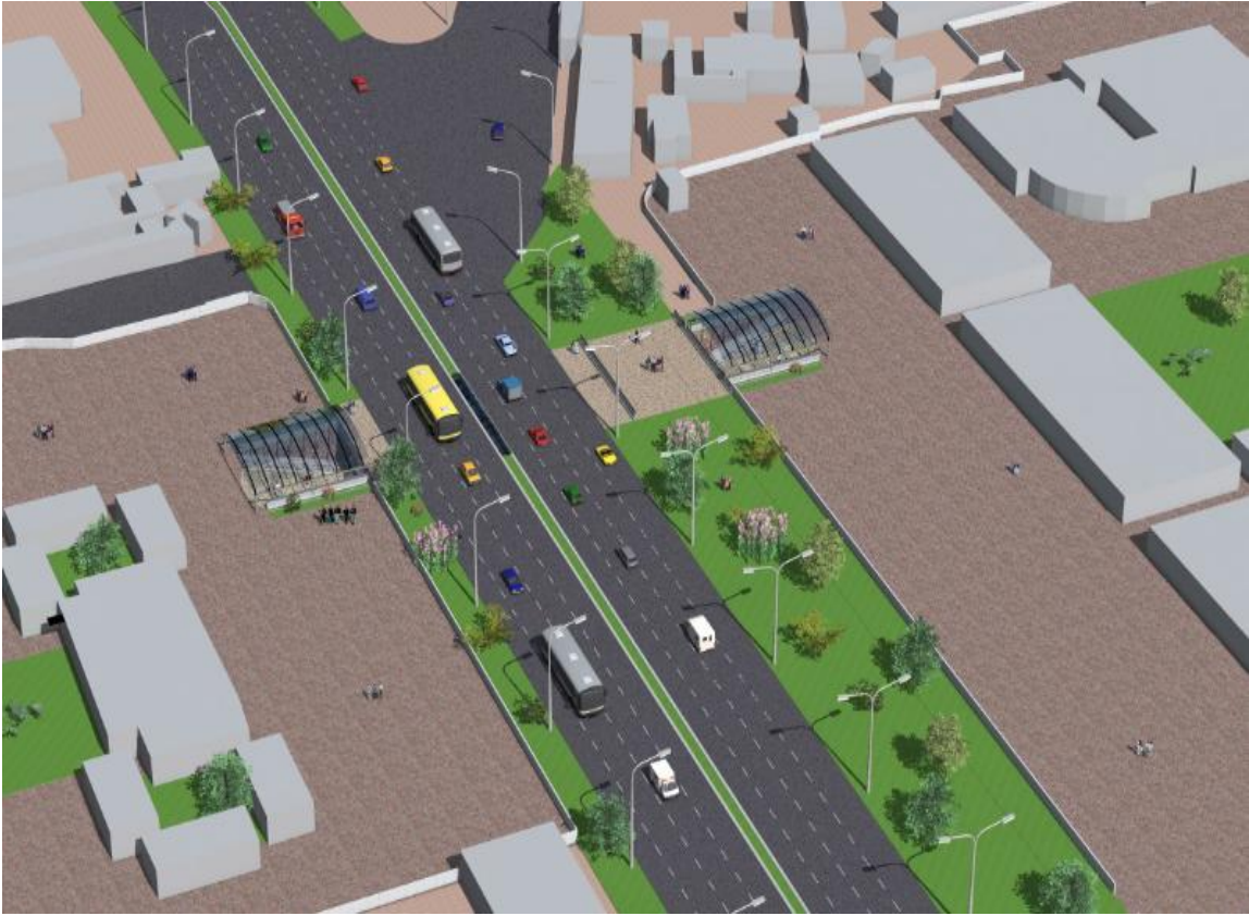
Picture 5-1: top view of the pedestrian underpass connecting the two campuses of Addis Ababa institute of Technology.
