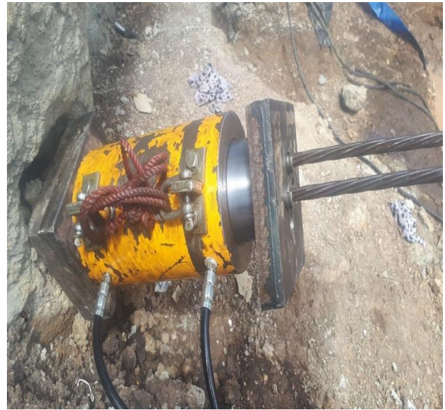
FIGURE 3-14 PLACING OF ANCHORAGE AND ANCHOR STRESS JACK TOOLS
