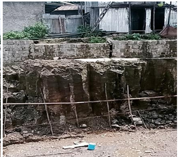
FIGURE 3-1 EXAMPLE OF EXCAVATION SUPPORT SYSTEM BY GRAVITY RETAINING WALL
