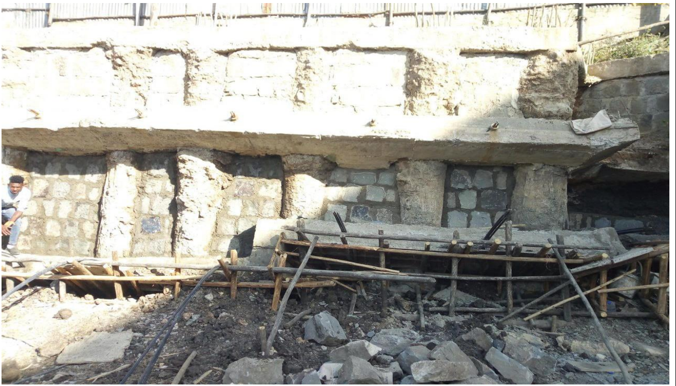
FIGURE 3-19 ANCHORED SHORING PILE WALL SYSTEM
