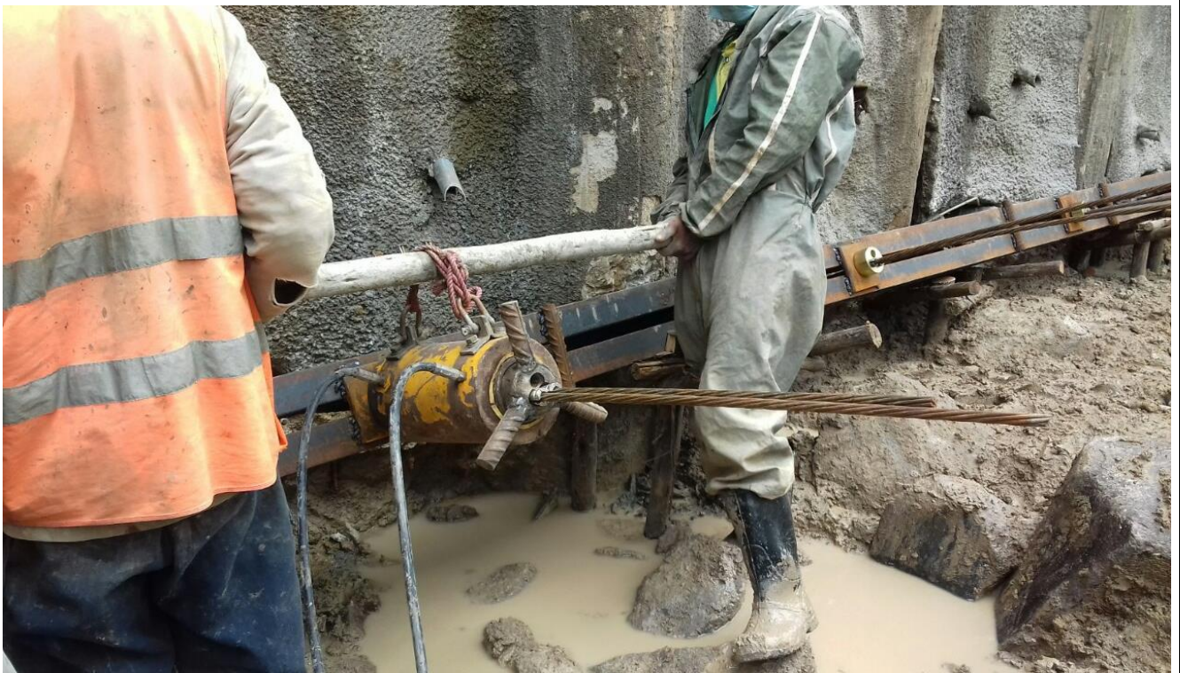
FIGURE 3-16 PLACING OF STEEL I-SECTION ANCHOR BEAM AND LOCKING OF ANCHOR
