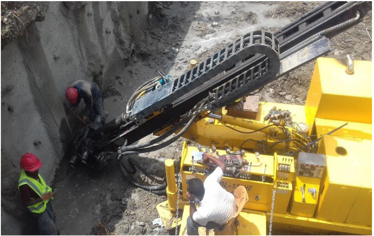
FIGURE 3-13 PILE CORE ANCHOR DRILLING
