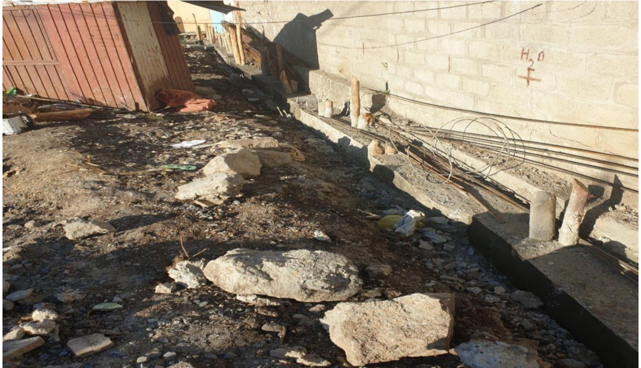
FIGURE 3-8 BRACING BEAM CONCRETE CASTING
