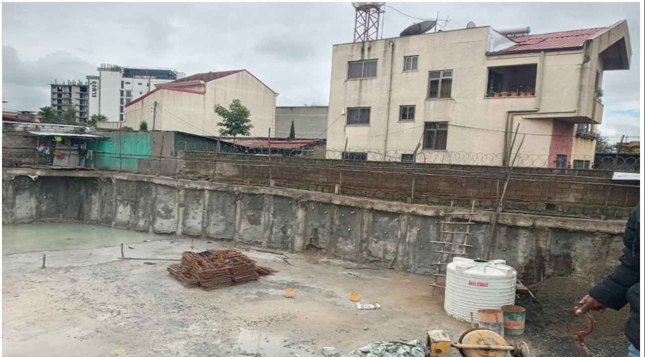
FIGURE 3-9 SHOTCRETE APPLICATION OF TIMBER PILE
