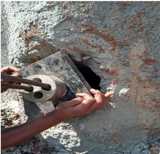
FIGURE 3-14 PLACING OF ANCHORAGE AND ANCHOR STRESS JACK TOOLS
