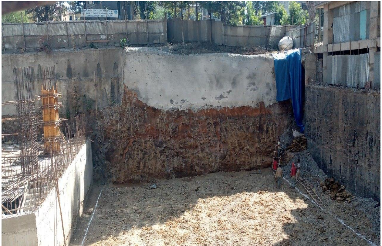
FIGURE 3-24 REINFORCEMENT SOIL NAILING WALL
