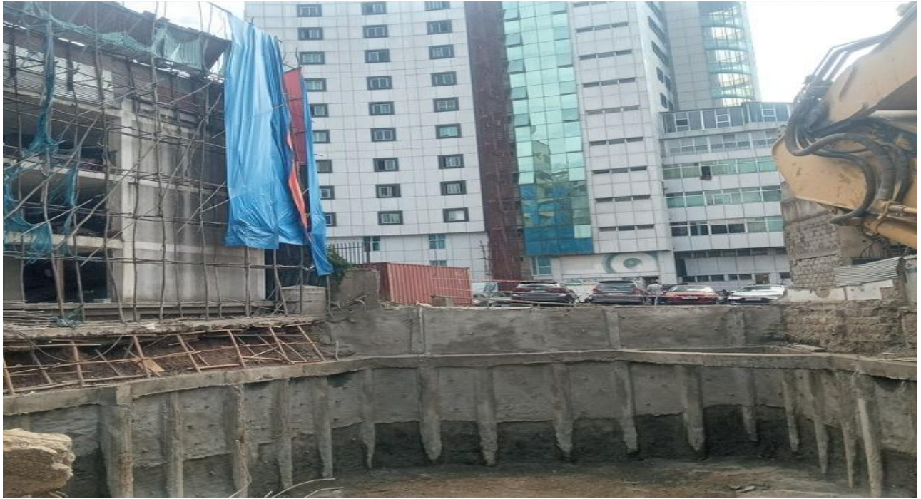
FIGURE 3-25 VIEW OF TOP SOIL NAILING WITH CONTIGUOUS PILE WALL SYSTEM
