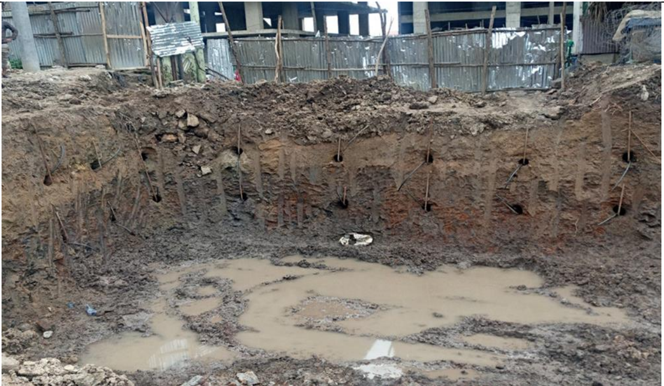
Figure 3-23 View of Soil Nailing Wall
