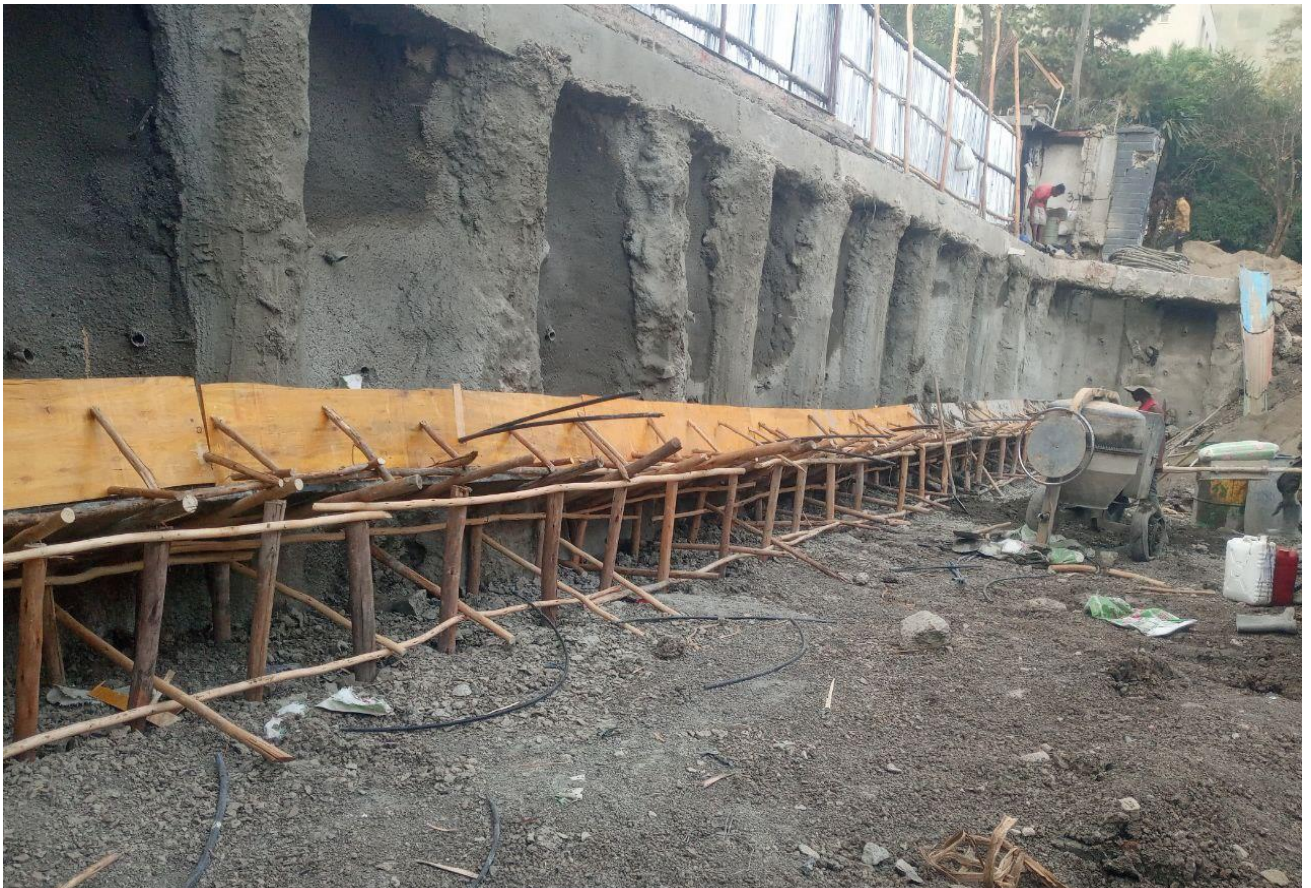
FIGURE 3-18 PREPARATION OF REBAR AND FORMWORK FOR RCC ANCHOR BEAM
