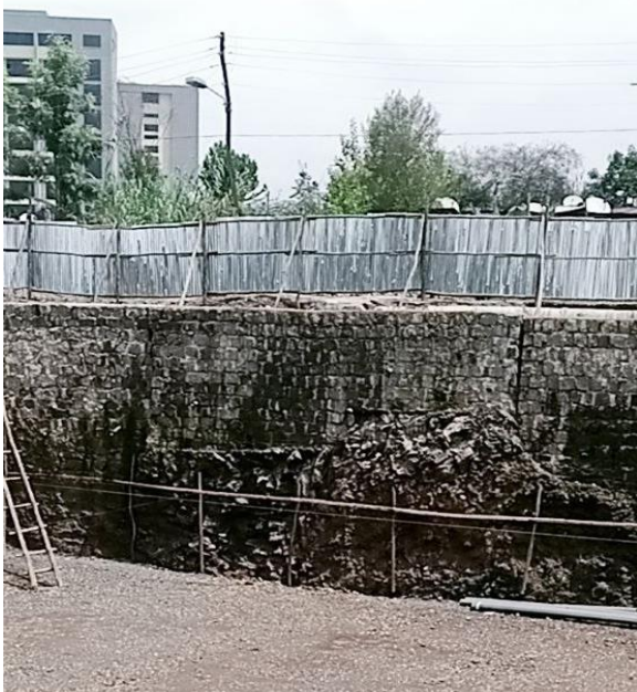
FIGURE 3-1 EXAMPLE OF EXCAVATION SUPPORT SYSTEM BY GRAVITY RETAINING WALL
