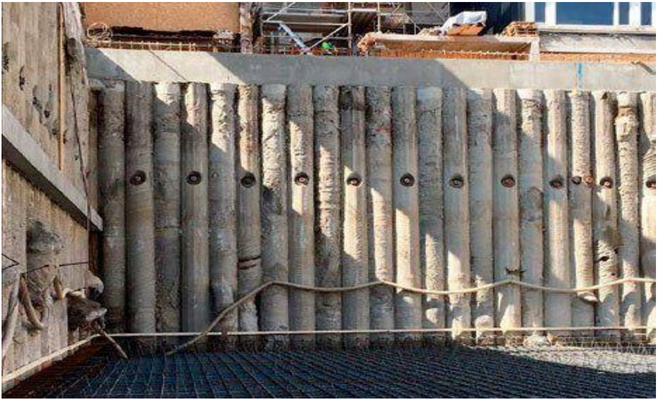
FIGURE 3-27 TANGENT PILE WALL
