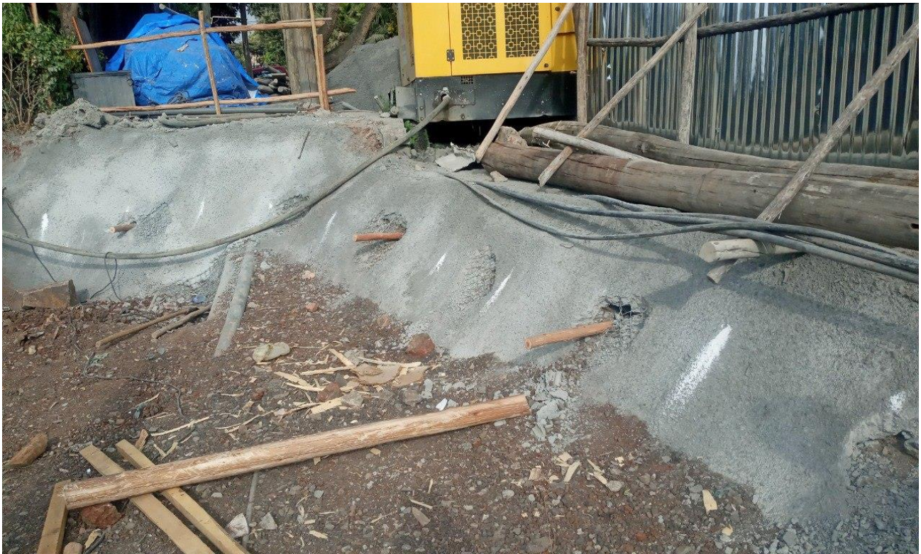
FIGURE 3-21 SOIL NAILING WITH TIMBER AND SHOTCRETE WALL
