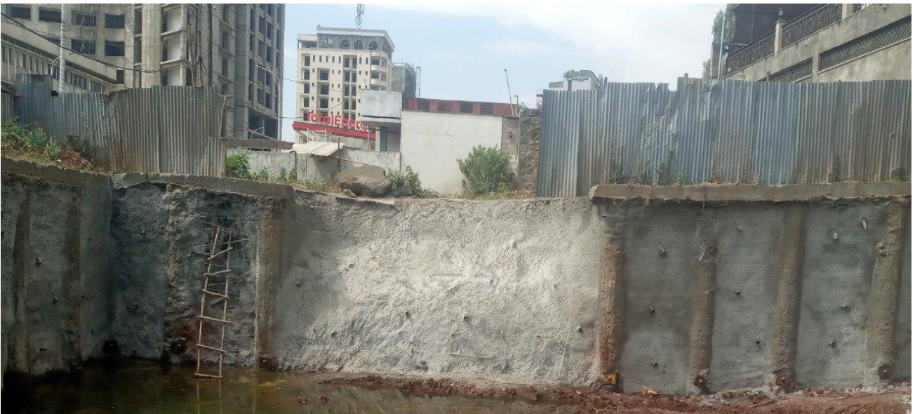
Figure 3-26 View of Soil Nailing Wall Between Contiguous Pile Wall Systems
