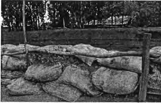
Figure 2. Flood dykes on the river Megech
