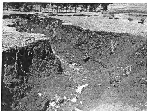
Gullies created by flooding
