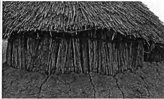
figure 3. A house built with raised platform, and Plastered with mud to protect from being flooded.
