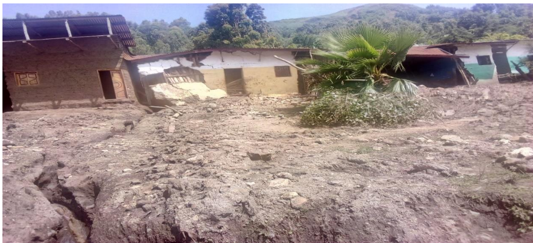
Figure 30: Homes destroyed by flooding in Amaya o1 village Konta Special District, SNNPR 2019
