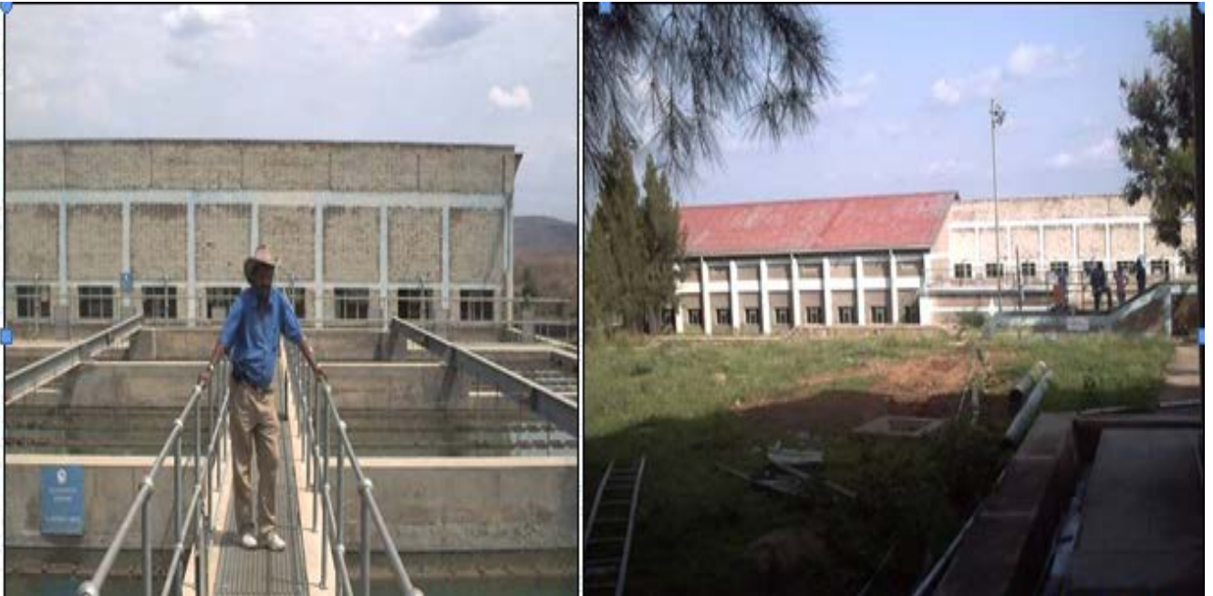
Plate No. 3-3 Partial View of Treatment Plant.
