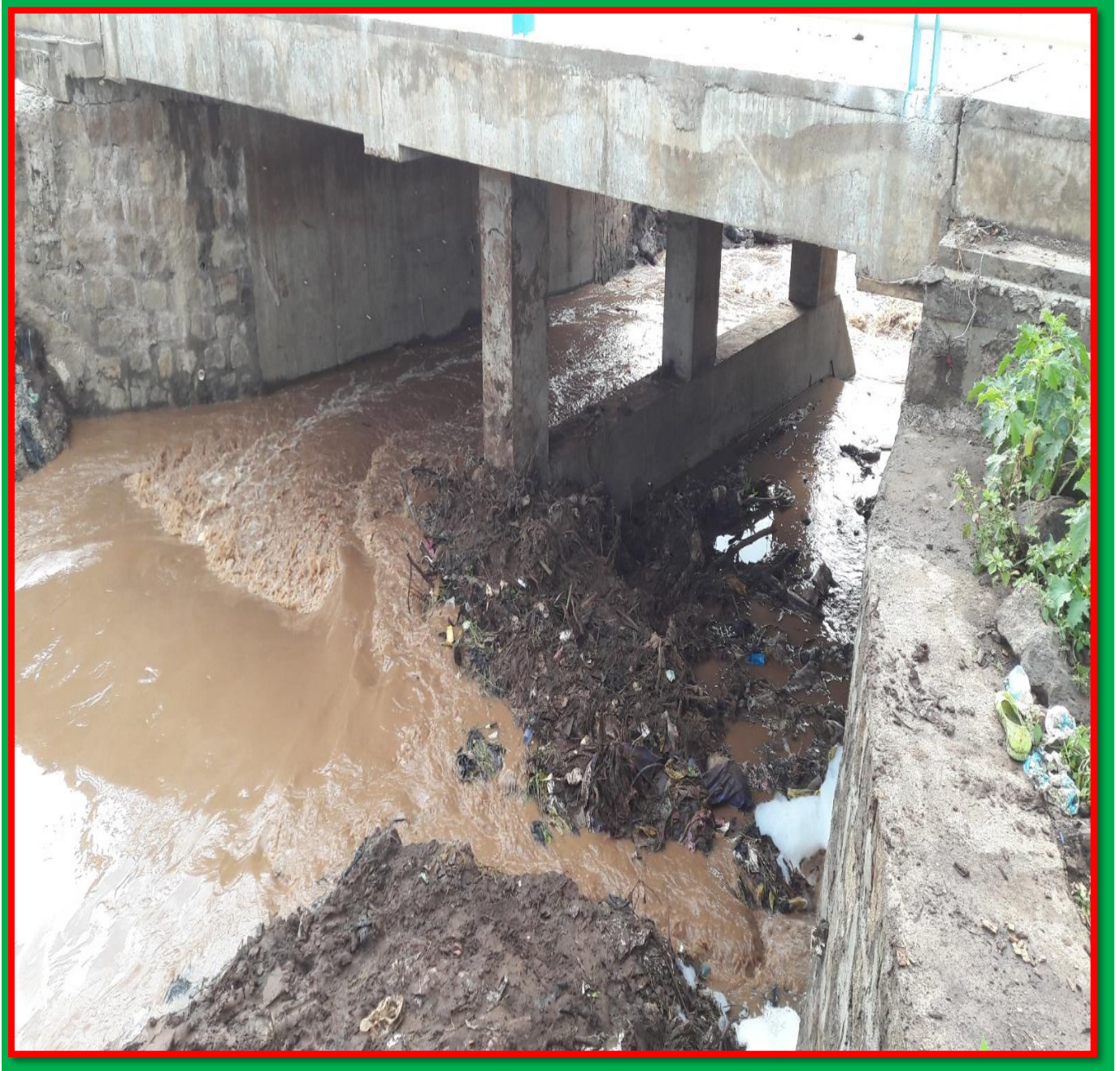
Figure 2-4: Urban storm water flooding and River pollution around weleta at D/S of Sebeta town
