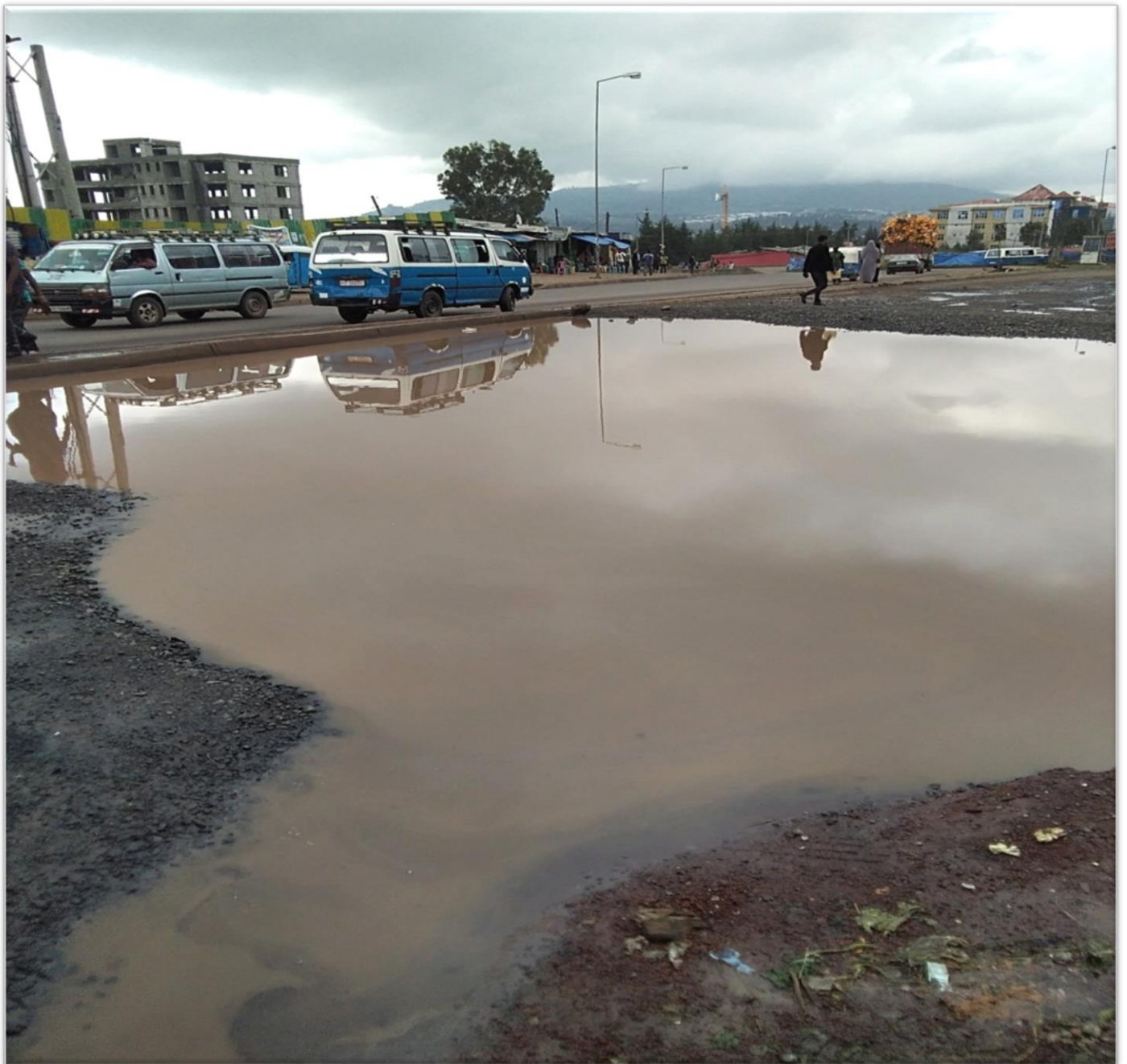
Figure 2-5: Effect of flood around waleta area road
