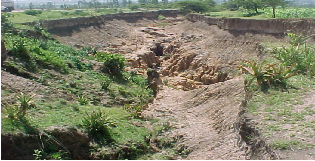
Plate 5.1 Deep Gully within Adilo River Catchment
