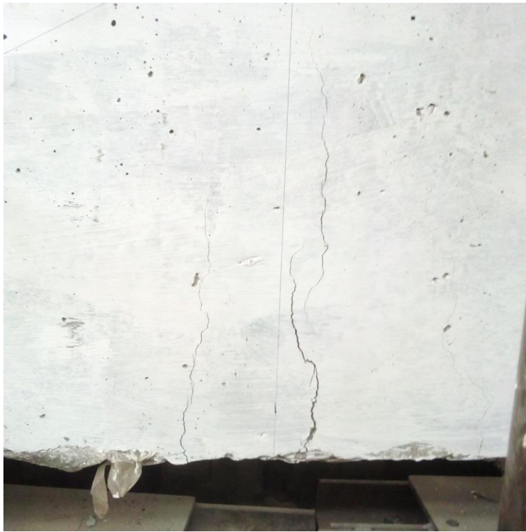
Figure 4-18 Early Mid span cracking before peak load SB-50
