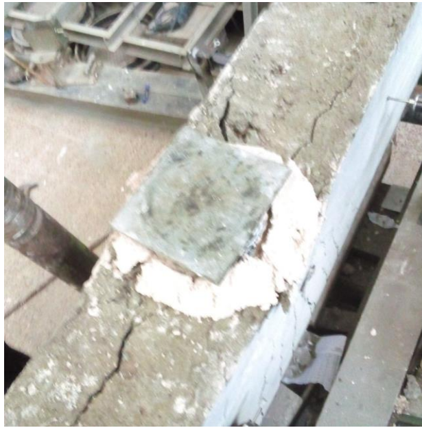
Figure 4-15 Final State of the Beam SA-75 top view
