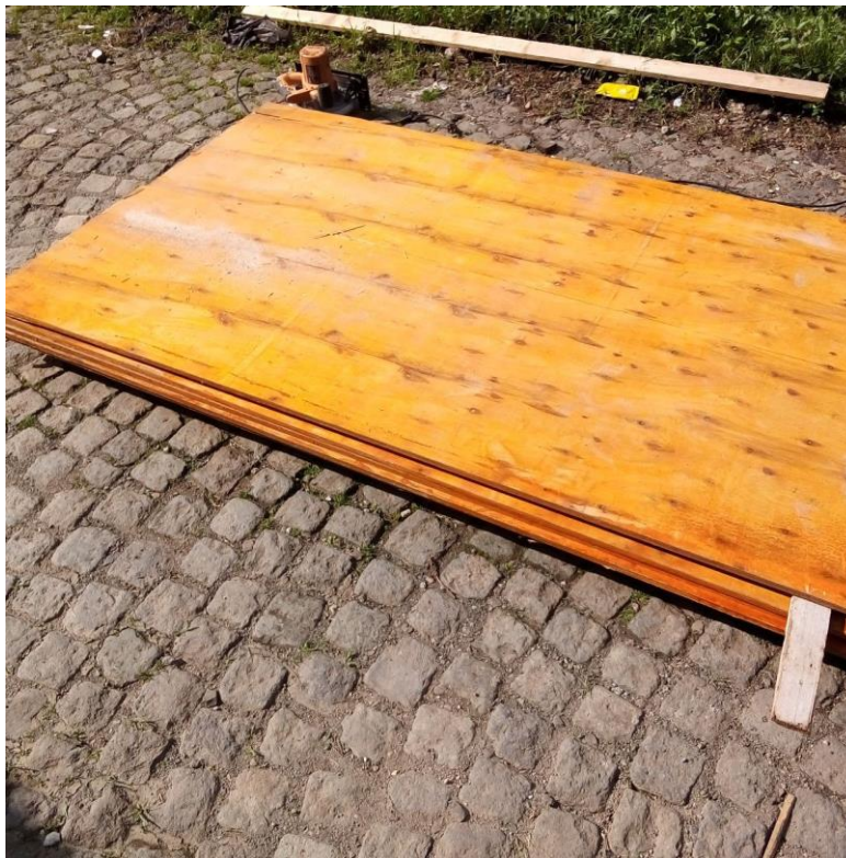
Figure 3-6 Plywood used for Formwork Construction
