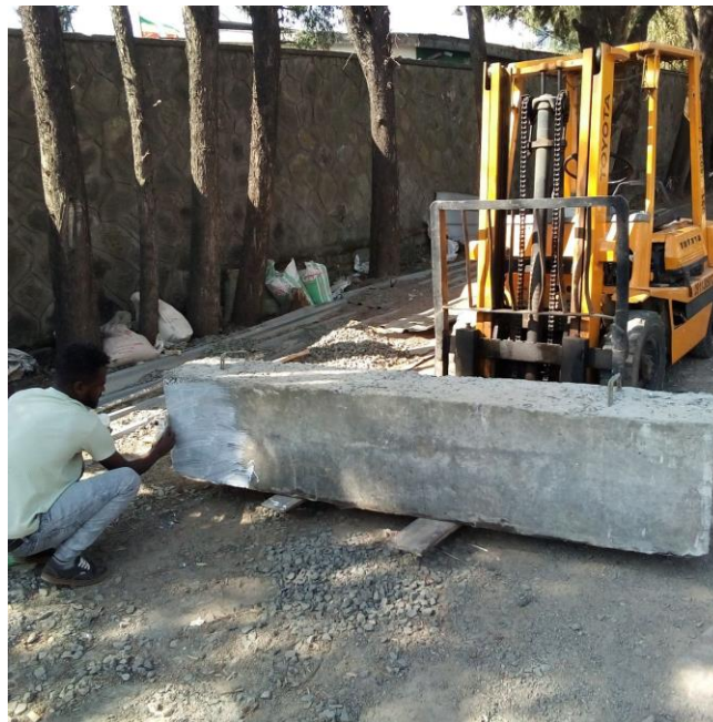
Figure 3-11 Getting ready the beams and transporting
