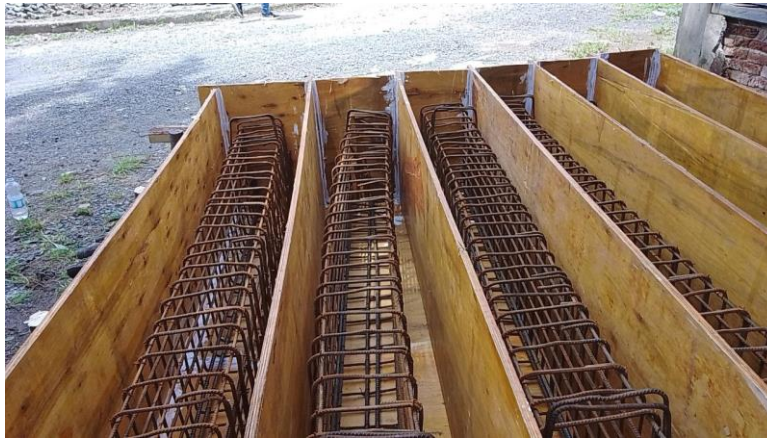
Figure 3-8 Reinforcement cages placed in the formwork
