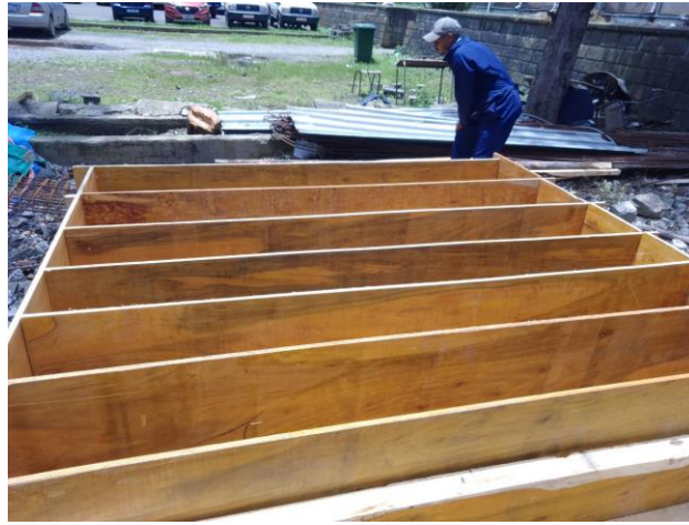
Figure 3-7 Formwork Assembly for Specimens
