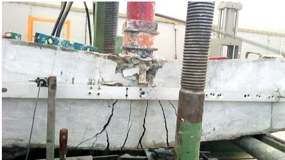
Figure 4-9 Spalling under load around peak load
