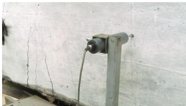
Figure 3-15 Displacement Transducer (For out of plane measurements)
