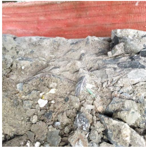
Figure 4-5 top of the beam after the test
