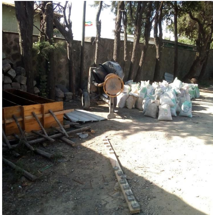
Figure 3-9 Materials and mixer ready for casting
