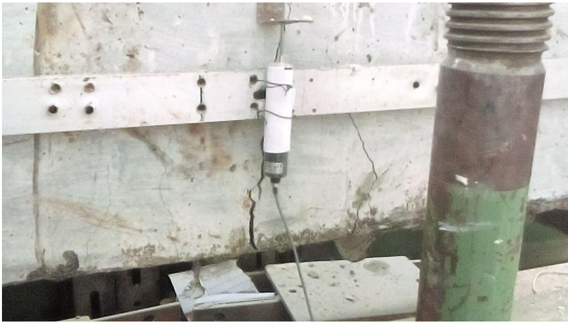
Figure 4-13 Mid span cracking before peak load SA-75
