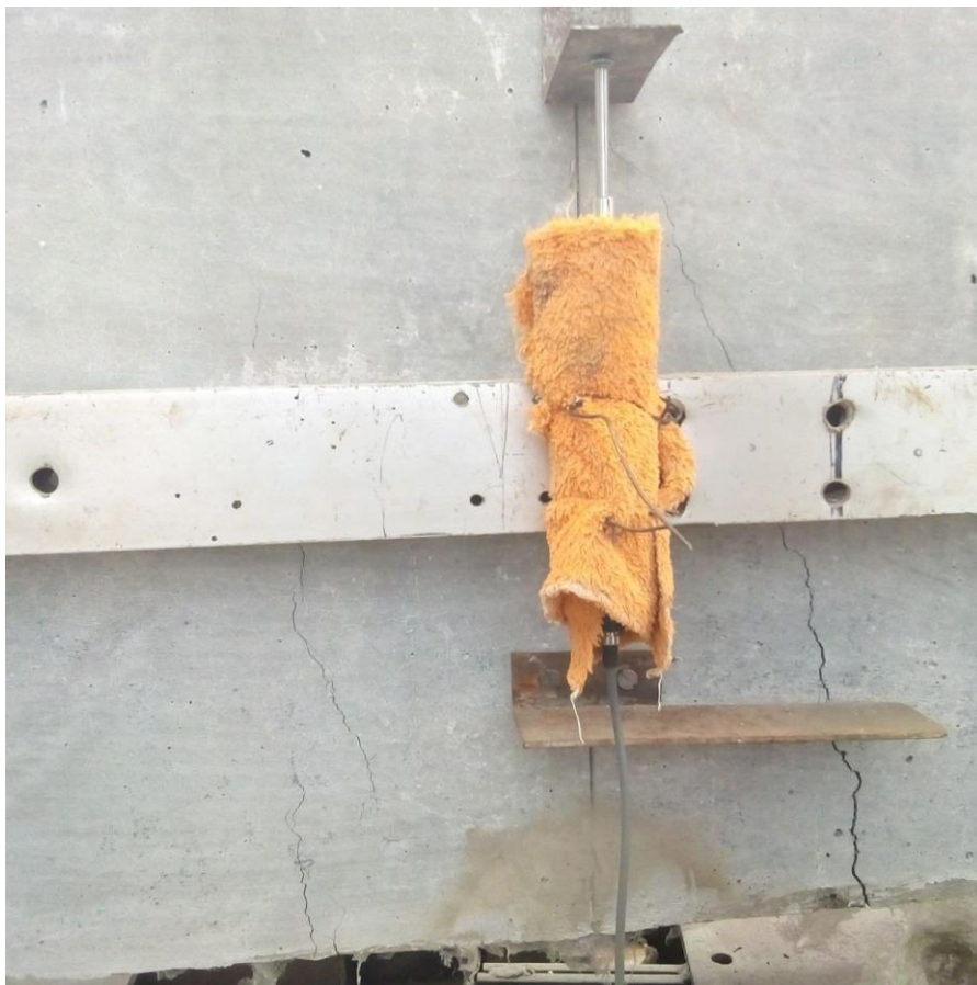
Figure 4-25 Early Mid span cracking before peak load SB-100
