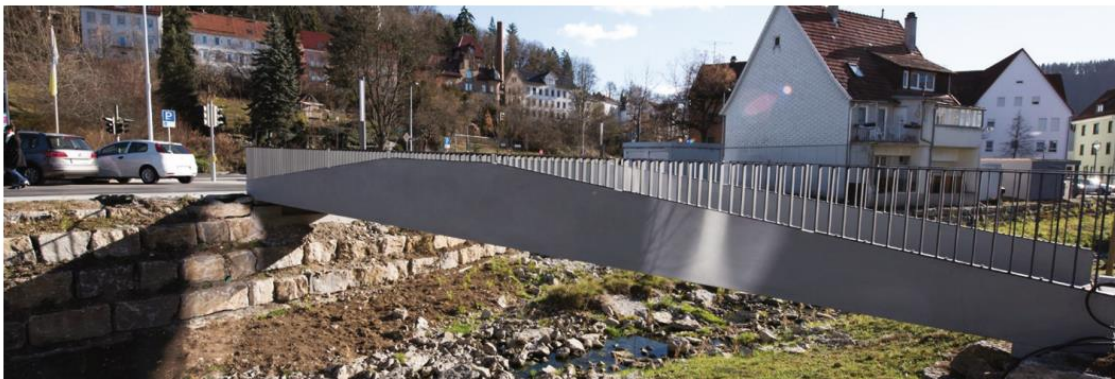
Figure 2-6 TRC pedestrian bridge in Albstadt, Germany (Rempel et al., 2018).
