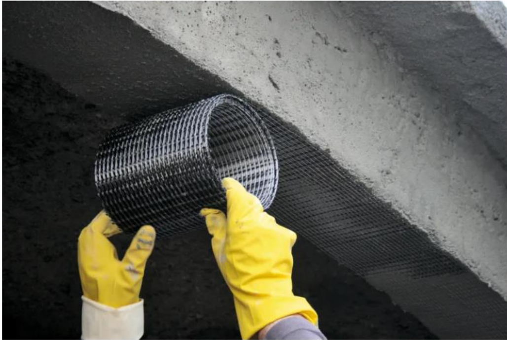
Figure 2-5 Hand lay-up TRC method for strengthened structure
