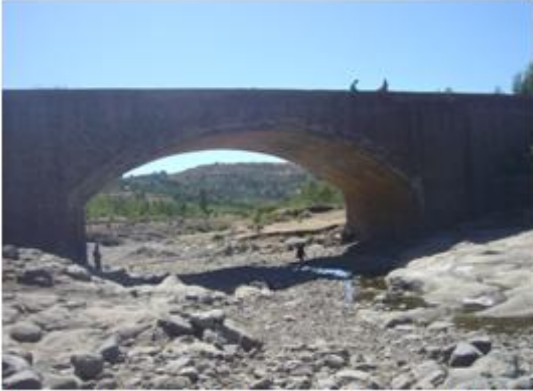
Figure 3.4 Angereb River Bridge
