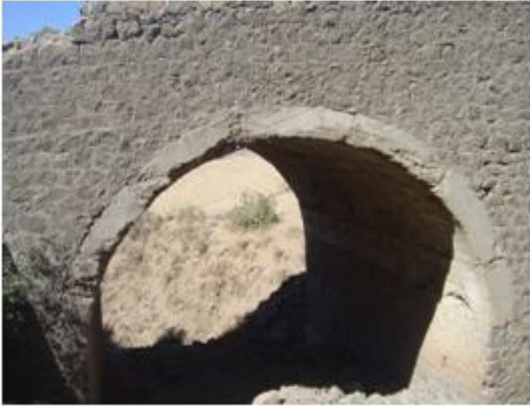
Figure 3.5 Amorageal River Arch Bridge
