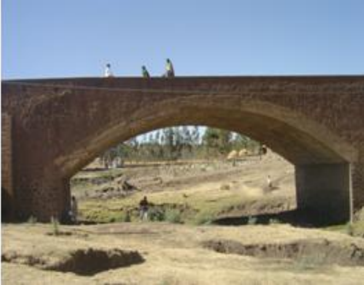
Figure 3.6 Alem Watch River Bridge
