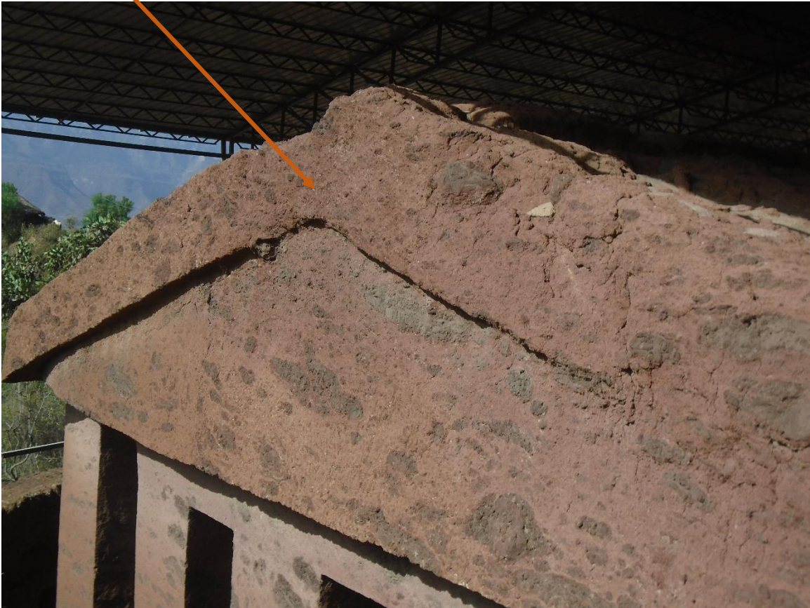
Figure36, Heavy roof of the church. (Source the author)
