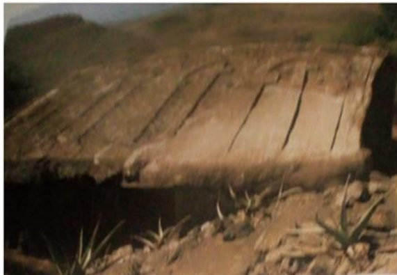
Damage of the rock due to bad restoration work.
