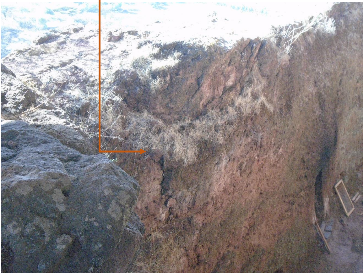
Figure18, The roof part of the church Betelhem (source the author.)
