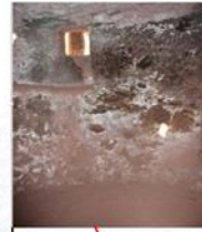
Damages due to water infiltration
