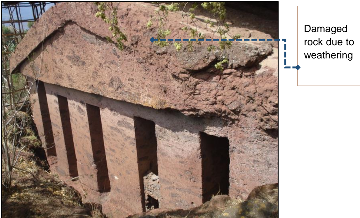
Figure 6: Damage Rock Due To Weathering (source the author)
