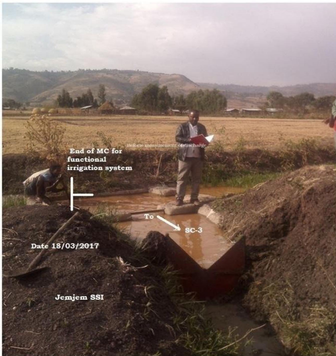
Figure B-6 canal flow before discharging over the weir during the measurement
