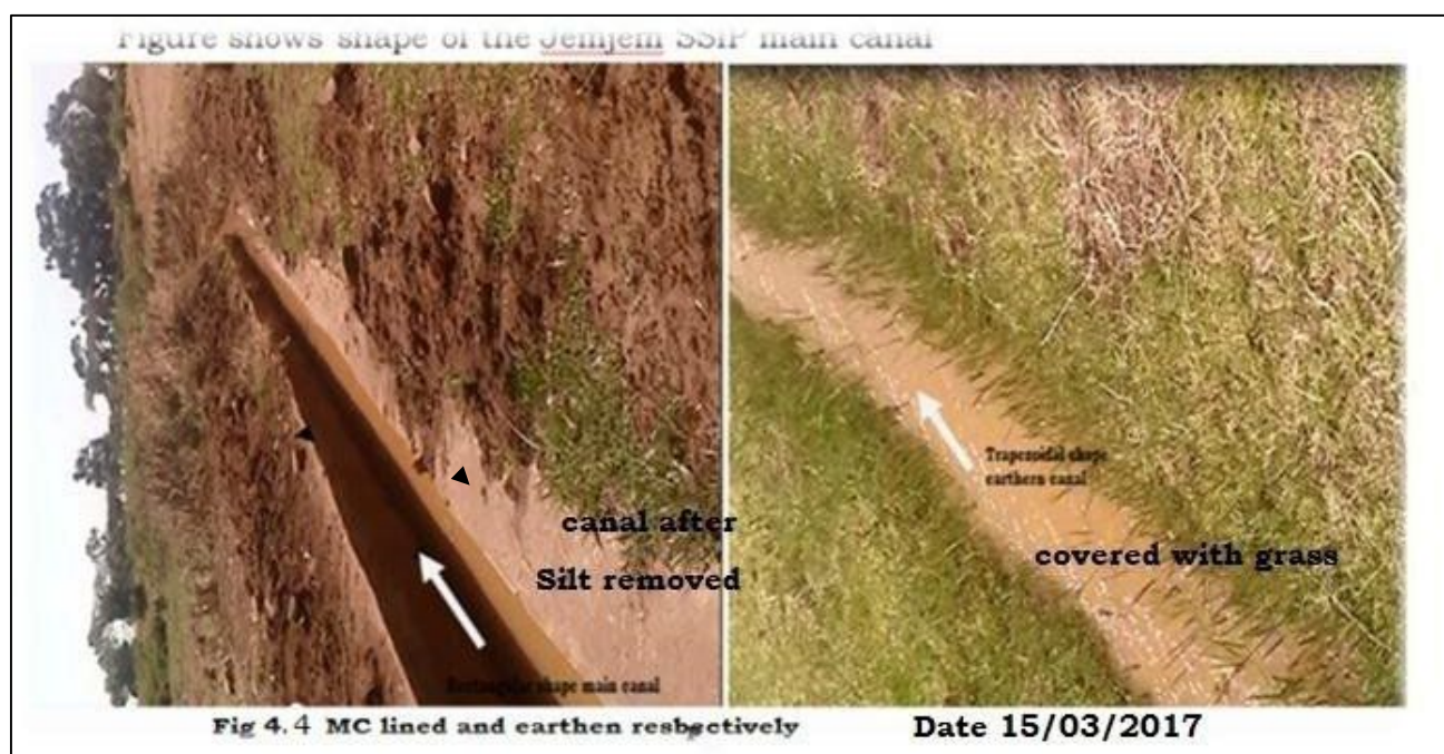
Figure 4.4 Desilted lined MC and earth canal covered with grass
