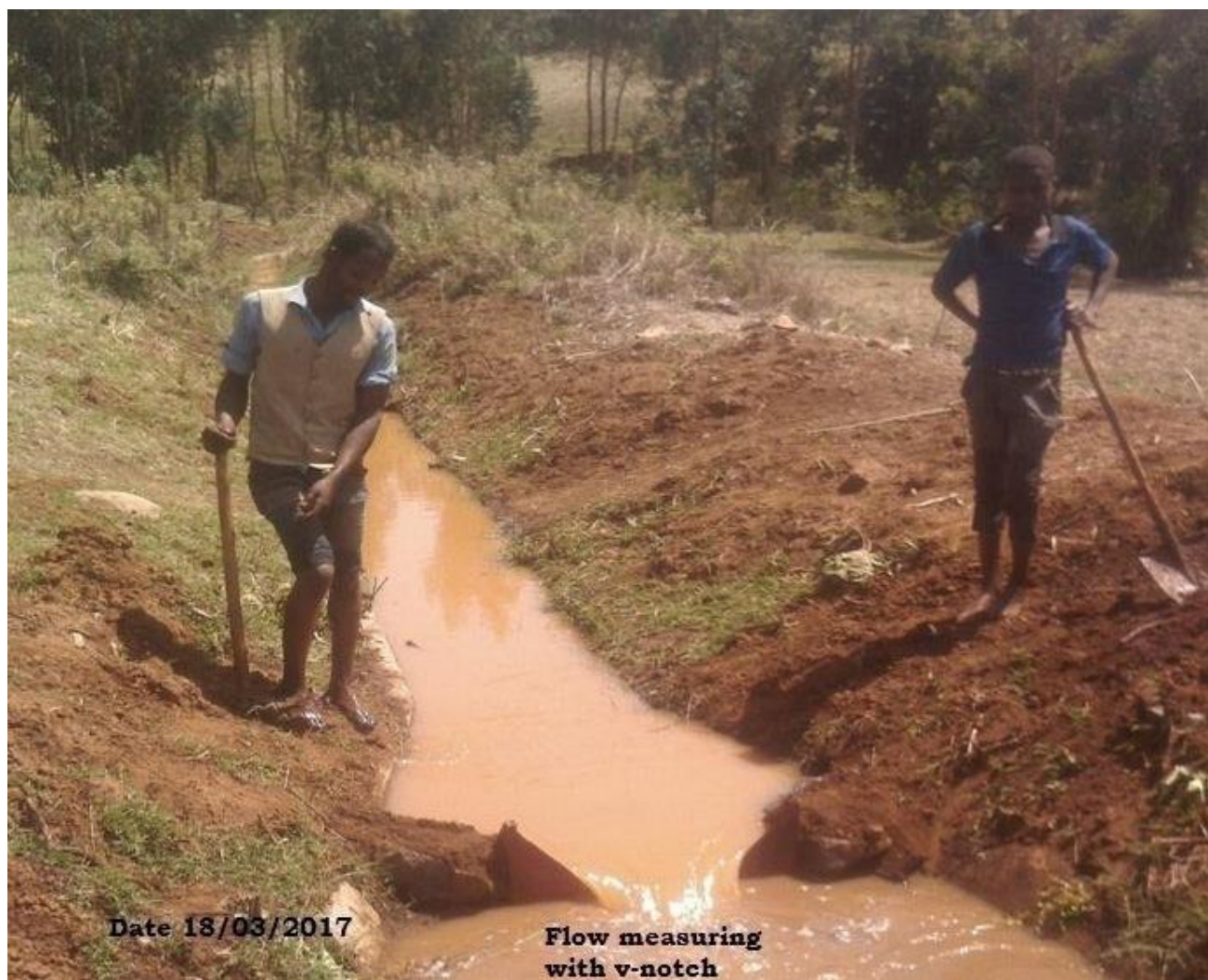
Figure B-2 Main canal discharge measurement of Jemjem SSI
