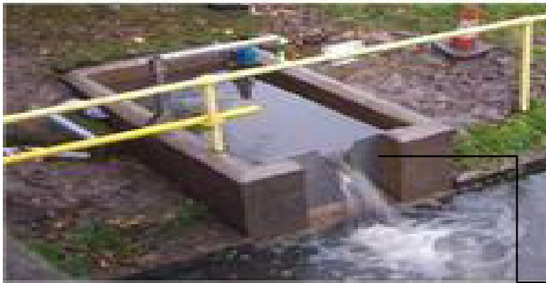
V Notch Weir
