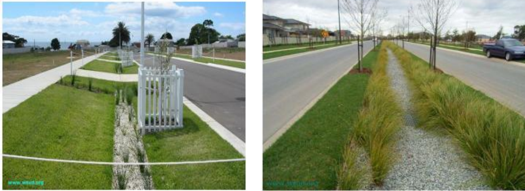
Fig. 5. 17: Grassed Swales (left) and Vegetated Swale (Right) ( Source: Water Sensitive Urban Design of the Sydney Region)
