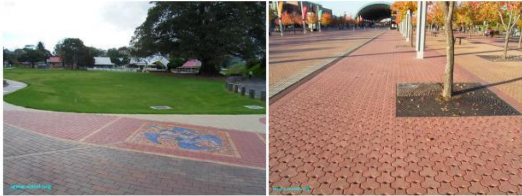
Fig.5.19a: Grassed Infiltration area (left) and Porous Paving (Right) ( Source: Water Sensitive Urban Design of the Sydney Region)
