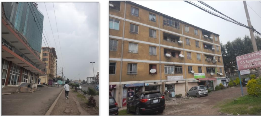
Figure 26 Existing Construction heights (source; Field survey, May 2023)
